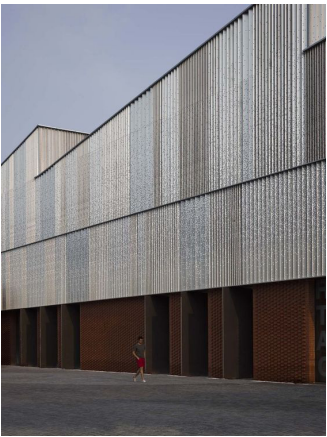
2 LIGHT CORRUGATED METAL PANEL LIGHT GRAY CORRUGATED ALUMINUM PANEL VERTICAL OR HORIZONTAL APPLICATION PER LOCATION
