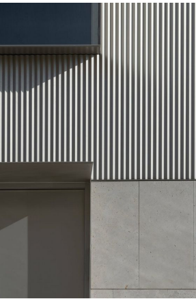
2 LIGHT CORRUGATED METAL PANEL LIGHT GRAY CORRUGATED ALUMINUM PANEL VERTICAL OR HORIZONTAL APPLICATION PER LOCATION
