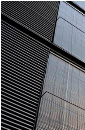
3 DARK CORRUGATED METAL PANEL CHARCOAL GRAY CORRUGATED ALUMINUM PANEL VERTICAL OR HORIZONTAL APPLICATION PER LOCATION
