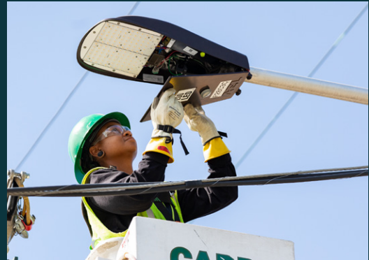
Local crew member installing new LED streetlight fixture
