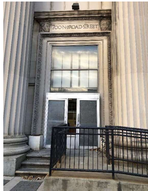
Figure 6. A view of the original main entrance. Original doors have been removed and infilled contemporary doors. An accessibility ramp has been added to the front of the building.
