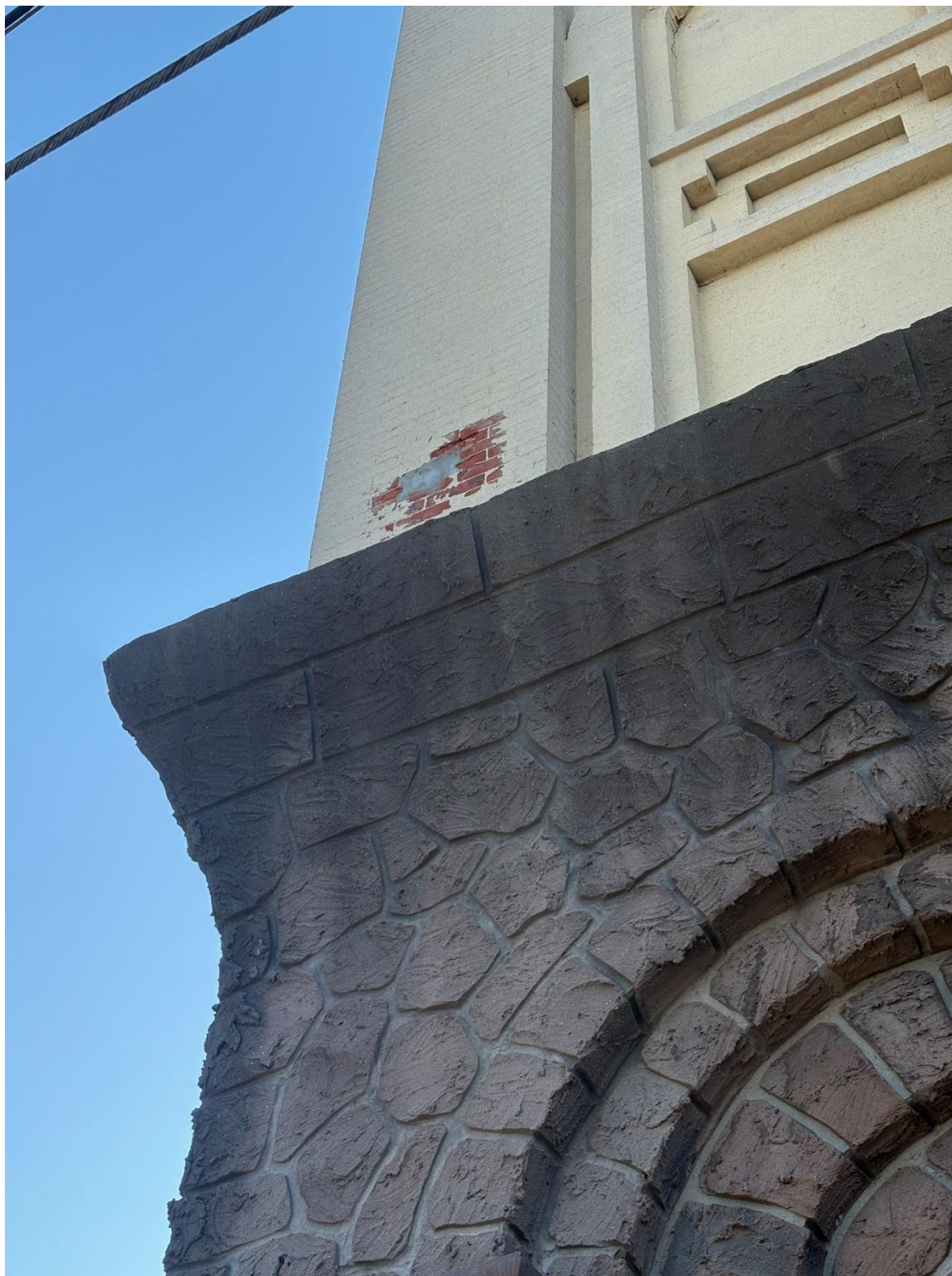
Image 7: The original brick is visible on the second and third elevations of the building. The original red brick is currently painted yellow. The first floor is currently clad in stone veneer.
