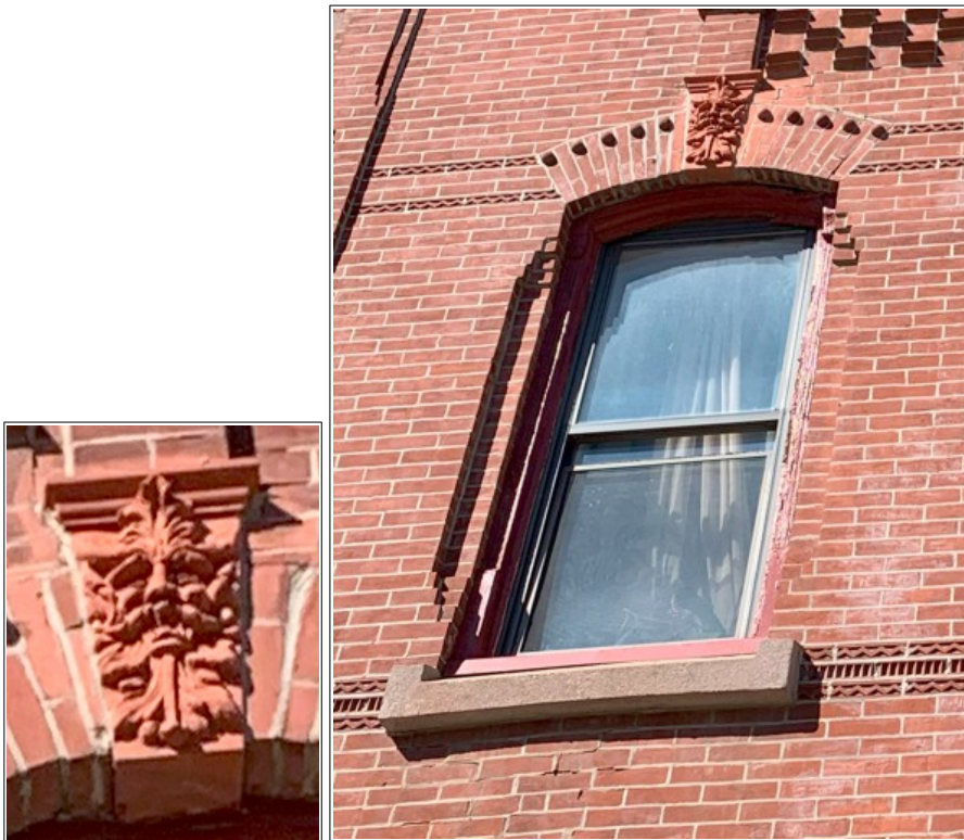
Figures 15, 16, and 17: The second-floor windows feature decorative arches using Peerless brick No. 10 and topped with a Green Man keystone.
