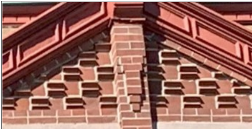
Figures 22 and 23: Detail showing the decoration on the gable adorned by a checkerboard pattern using the No. 25 brick.
