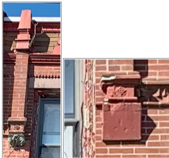
Figures 46 and 47: Two smaller pilasters flank the windows. The left pilaster is relatively intact while the bottom bracket of the one on the right has been replaced by a simpler concrete element.
