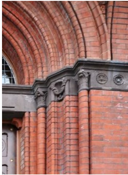
Figure 91: Entrance Detail showing the “rich mouldings of beads, coves, fillets, angles and quirks” created with Peerless bricks.
