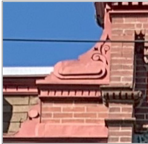
Figures 39 and 40: A protruding course of somewhat deteriorated notched brick, style 135, aligns with a notched band that echoes the design of the parapet wall cornice behind it. Two pairs of sloped panels (the larger one incised with a curved decoration) soften the transition between setbacks.
