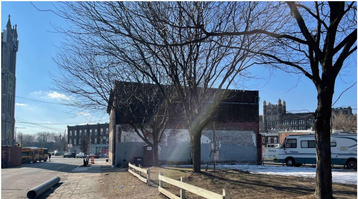
FIGURE 10: Rear (north) elevation of the building, looking from Lancaster Avenue, showing "ghost lines" of former attached structures. (PC, typ. all pics)
