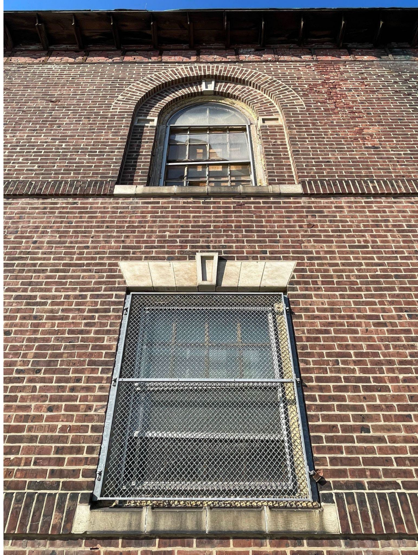
FIGURE 6: East elevation, showing typical ground level rectangular “splayed lintel” windows, and second level (“piano nobile”/noble floor reminiscent) with arched windows inset into concentric relieving arches and decorative carved relief keystones. These are found on both east and west elevations in sets of three. (PC)
