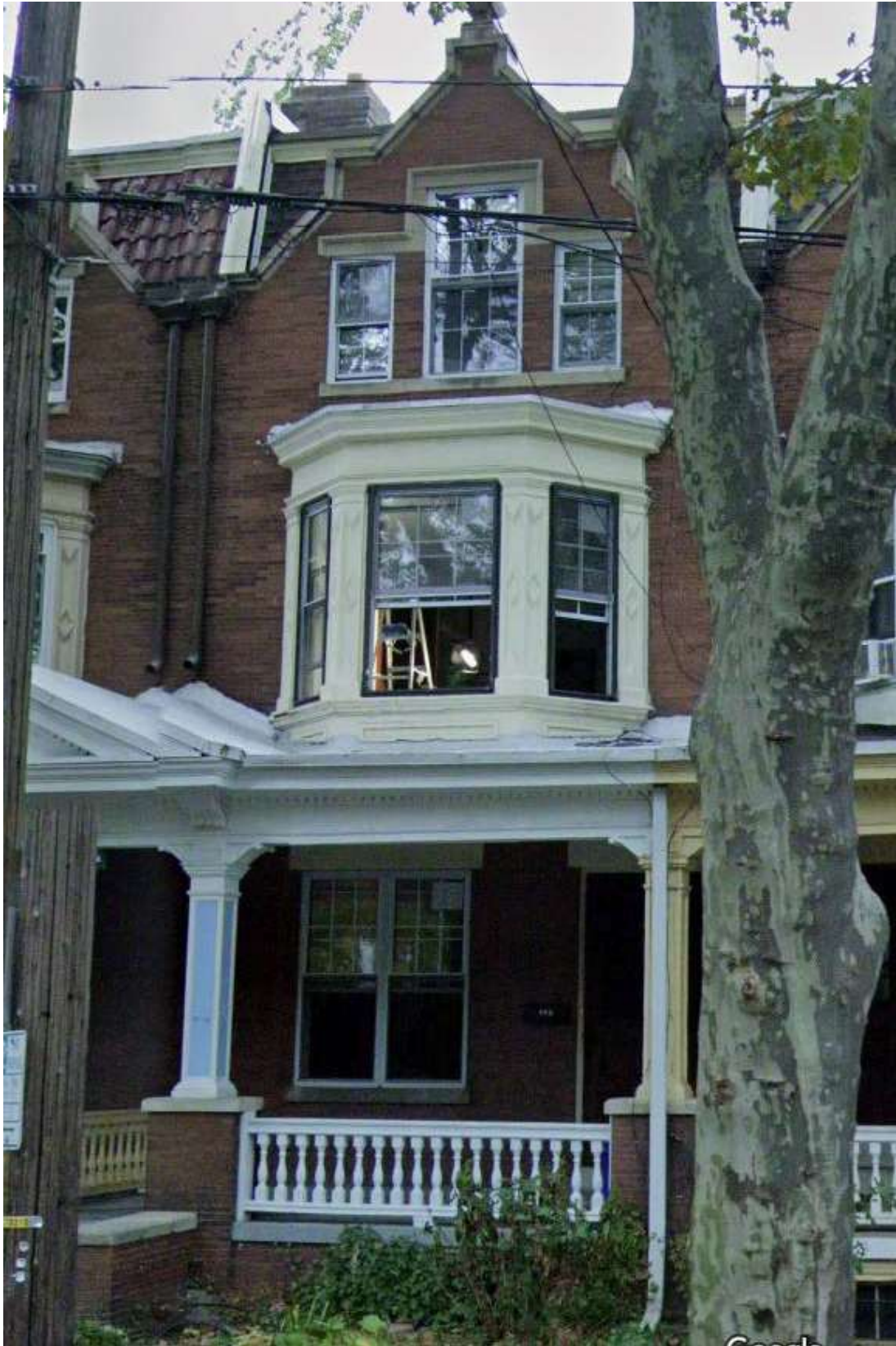
Figure 2. 327 N 34 th Street, 2024. Front façade showing vinyl replacement windows. Image source: Google Streetview.
