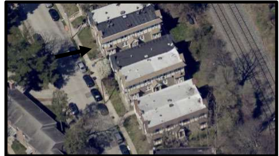
Top: The southwest and southeast elevations. Source: Oscar Beisert, 2025. Middle: The southwest elevation. Source: Oscar Beisert, 2025. Bottom: Looking north, this aerial view depicts the subject property in context. Source: EagleView, March-April 2024, Atlas, City of Philadelphia.
