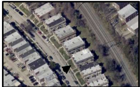
Top: The southwest and southeast elevations. Source: Oscar Beisert, 2025. Middle: The southwest elevation. Source: Oscar Beisert, 2025. Bottom: Looking north, this aerial view depicts the subject property in context. Source: EagleView, March-April 2024, Atlas, City of Philadelphia.
