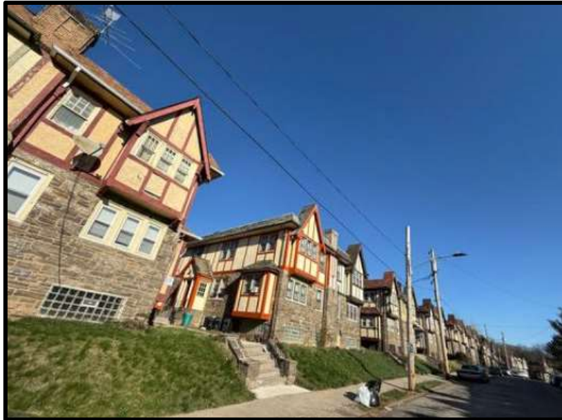
Figure 7. Top: Looking southeast, the view of the terrace of twin apartment houses that comprises the district from the frontage of 6655 Blakemore. Figure 8. Bottom: Looking southeast at the row of twin apartment houses that form the district. Source: Oscar Beisert, 2025.
