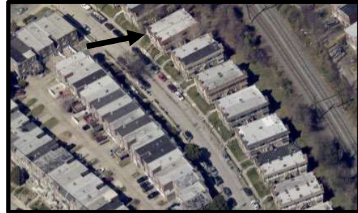
Top: The northwest and southwest elevations. Source: Oscar Beisert, 2025. Middle: The northwest and southwest elevations. Source: Oscar Beisert, 2025. Bottom: Looking north, this aerial view depicts the subject property in context. Source: EagleView, March-April 2024, Atlas, City of Philadelphia.
