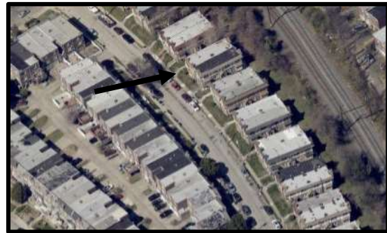
Top: The northwest and southwest elevations. Source: Oscar Beisert, 2025. Middle: The southwest elevation. Source: Oscar Beisert, 2025. Bottom: Looking north, this aerial view depicts the subject property in context. Source: EagleView, March-April 2024, Atlas, City of Philadelphia.
