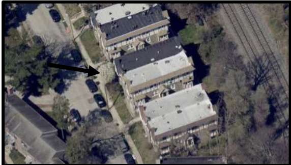
Top: The northwest and southwest elevations. Source: Oscar Beisert, 2025. Middle: The southwest elevation. Source: Oscar Beisert, 2025. Bottom: Looking north, this aerial view depicts the subject property in context. Source: EagleView, March-April 2024, Atlas, City of Philadelphia.
