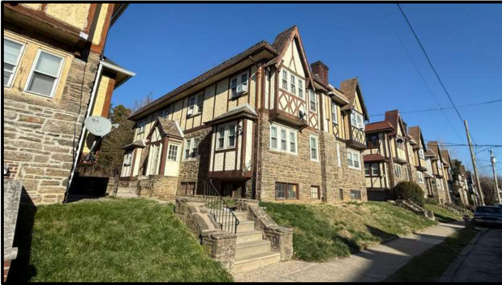
Figure 1. Looking north, the lower end of the buildings that comprise the subject historic district. Figure 2. Looking northeast, the courtyard and street-facing elevations. Source: Oscar Beisert, 2025.
