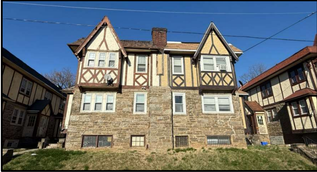
Figure 28. The southeast elevation of 6629 (on right) and 6631 (on left) Blakemore, showing a more decorative example of the Tudor Revival half timbering within the second floor details. Source: Oscar Beisert, 2025.
