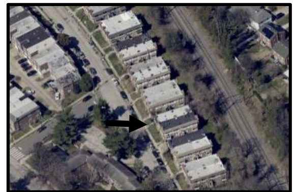
Top: The southwest elevation. Source: Oscar Beisert, 2025. Middle: The southwest and northwest elevations. Source: Oscar Beisert, 2025. Bottom: Looking north, this aerial view depicts the subject property in context. Source: EagleView, March-April 2024, Atlas, City of Philadelphia.
