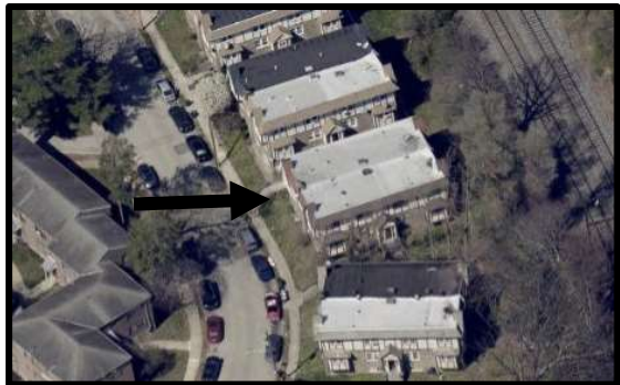
Top: The southwest elevation. Source: Oscar Beisert, 2025. Middle: The northwest and southwest elevations. Source: Oscar Beisert, 2025. Bottom: Looking north, this aerial view depicts the subject property in context. Source: EagleView, March-April 2024, Atlas, City of Philadelphia.
