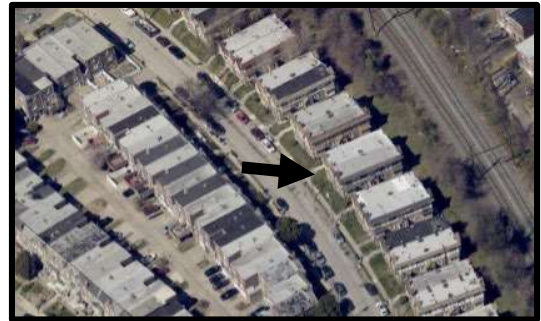
Top: The northwest and southwest elevations. Source: Oscar Beisert, 2025. Middle: The southwest elevation. Source: Oscar Beisert, 2025. Bottom: Looking north, this aerial view depicts the subject property in context. Source: EagleView, March-April 2024, Atlas, City of Philadelphia.
