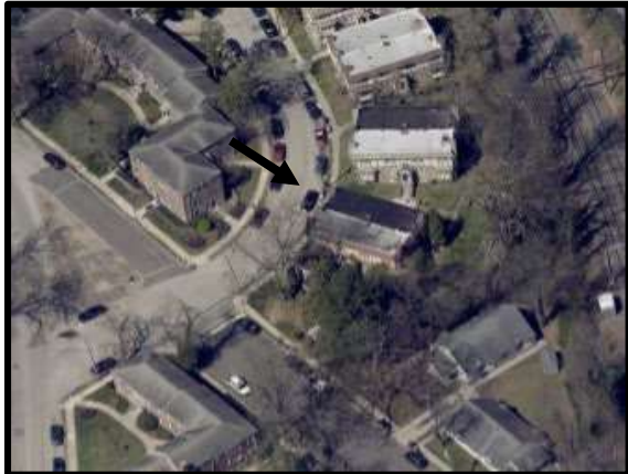
Top: The northeast and northwest elevations. Source: Oscar Beisert, 2025. Middle: The northeast elevation. Source: Oscar Beisert, 2025. Bottom: Looking north, this aerial view depicts the subject property in context. Source: EagleView, March-April 2024, Atlas, City of Philadelphia.
