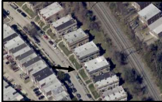
Top: The northwest and southwest elevations. Source: Oscar Beisert, 2025. Middle: The southwest elevation. Source: Oscar Beisert, 2025. Bottom: Looking north, this aerial view depicts the subject property in context. Source: EagleView, March-April 2024, Atlas, City of Philadelphia.
