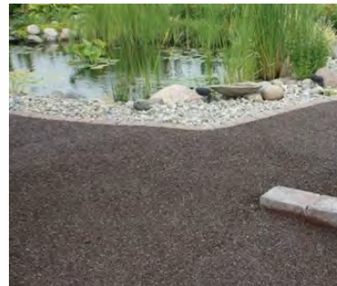
Resin-bound aggregate paving
