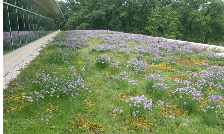
Extensive (shallow) green roof planting
