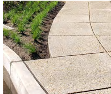
Exposed Aggregate Conc.
