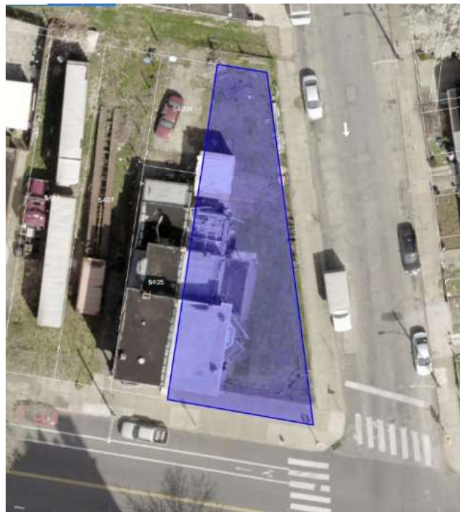
Figure 1. Aerial photo of 5401-03 Vine Street, Philadelphia, PA showing the lot boundaries. Vine Street appears at the bottom of the image and 54 th Street to the right. Image from Atlas.phila.gov.
