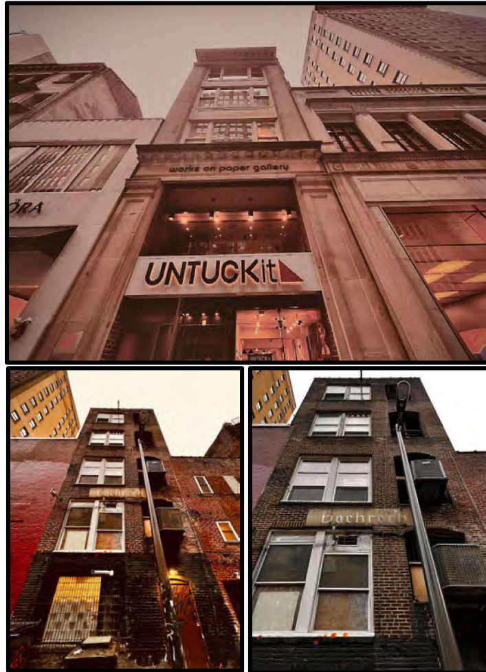
Figure 5. Top: Looking upward at the details within the primary (south) elevation. Figure 6. Bottom left: The rear (north) elevation of the subject property. Figure 7. Right: The rear (north) elevation of the subject property. Source: Oscar Beisert, 2022.
