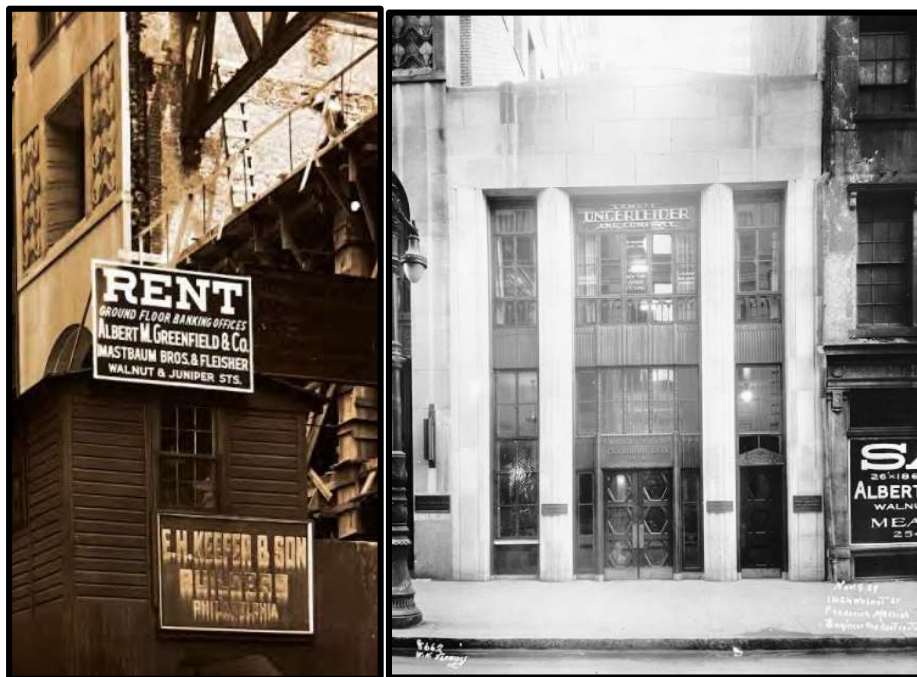
Figure 24. Left: The trend of commissioning new rental buildings in the 1400, 1500, and 1600 blocks of Walnut Street for potential banking and brokerage houses continued through 1929, as illustrated in this photo related to the construction of a new structure at 1424 Walnut Street (shown in Figure 23). As is visible construction was underway even before a tenant had been found for the ground floor, involving both Albert M. Greenfield & Co. and Mastbaum Brothers & Fleisher. Figure 25. Right: At the time of completion, the tenants included both Goodbody & Co. on the ground floor and Samuel Ungerleider and Company on the upper floor. Source: The Frederick and Edith L. Massiah Papers were donated to the University of Pennsylvania Archives by Louis J. Massiah in August 2011 (Accession # 2011:048).
