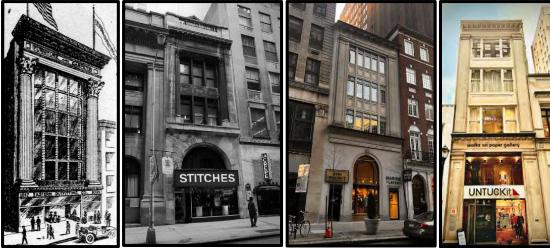
Figure 26. Left: The Eastern Outfitting Company (1909) at 1017-19 Market Street in San Francisco, California. Source: Grand Illusion - FoundSF . Figure 27. Middle left: The Republican Trust Company at 1429 Chestnut Street. Figure 28. Middle right: 1604 Walnut Street. Source: Oscar Beisert, 2022. Figure 29. Right: The subject property. Source: Oscar Beisert, 2022.
