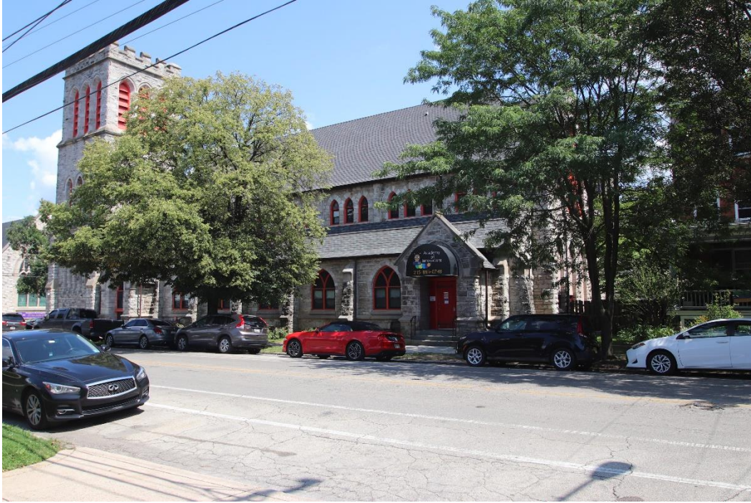
Photo 2: Church of the Atonement, northwest elevation. looking east. (Adrian Trevisan, 2023)
