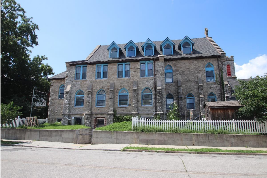
Photo 7: Parish House, southeast elevation, looking northwest. (Adrian Trevisan, 2023)
