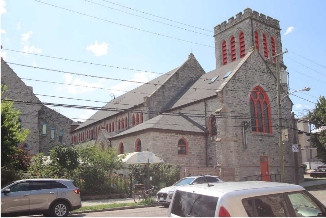
Photo 4: Church of the Atonement, northeast elevation, looking west. (Adrian Trevisan, 2023)
