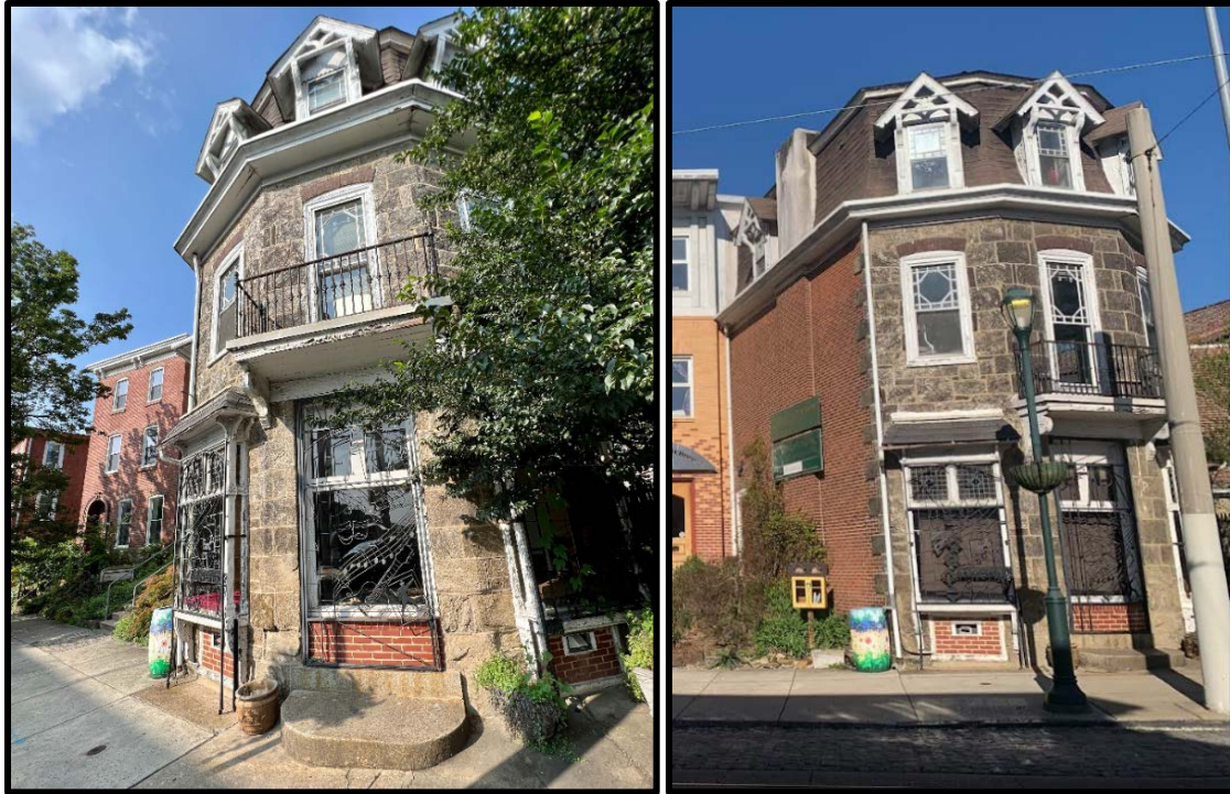
Figure 3 Left: The primary elevation (southwest) elevation of 6519 Germantown Avenue Source: Keeping Society of Philadelphia, 2023. Figure 4. The side (northwest) and primary (southwest) elevations of 6519 Germantown Avenue. Source: Keeping Society of Philadelphia, 2023.
