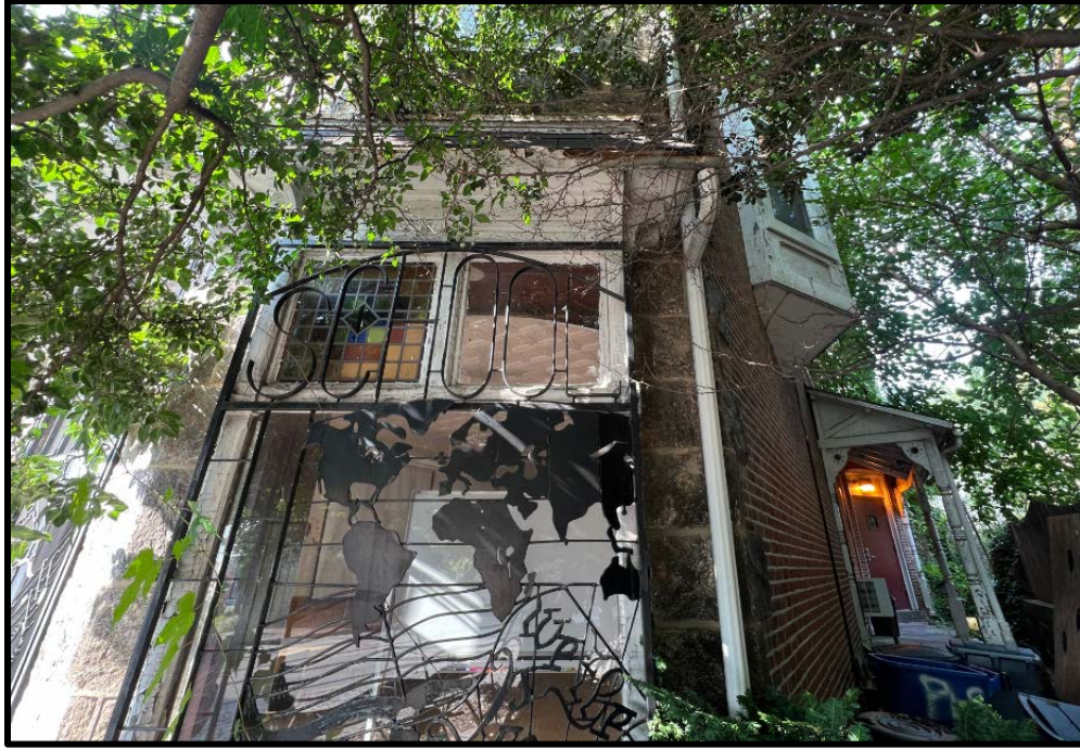
Figure 5. The southerly shop window within the Wissahickon schist façade and the side (southeast) elevation with the bay window above on the second floor and the side porch. Source: Keeping Society of Philadelphia, 2023.
