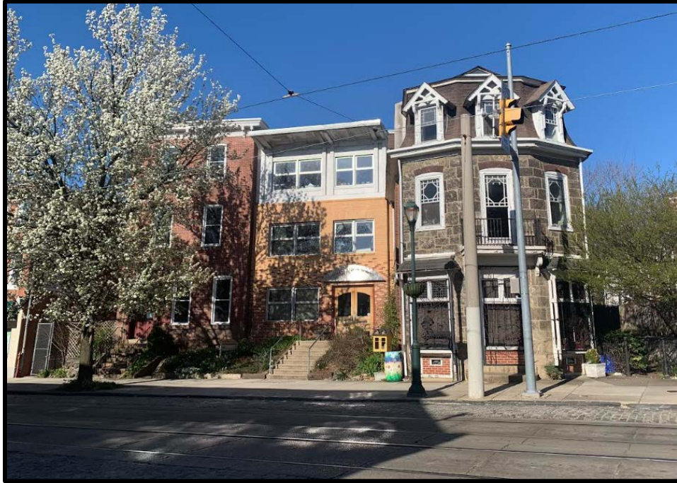
Figure 1. The primary (southwest) elevation of the subject property. Source: Keeping Society of Philadelphia, 2022.
