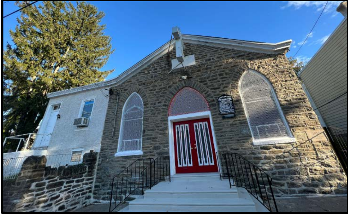
Figure 3. Grace Baptist Church, 34-36 E. Sharpnack Street, Primary (Northwest) Elevations. Source: Oscar Beisert, 2024.
