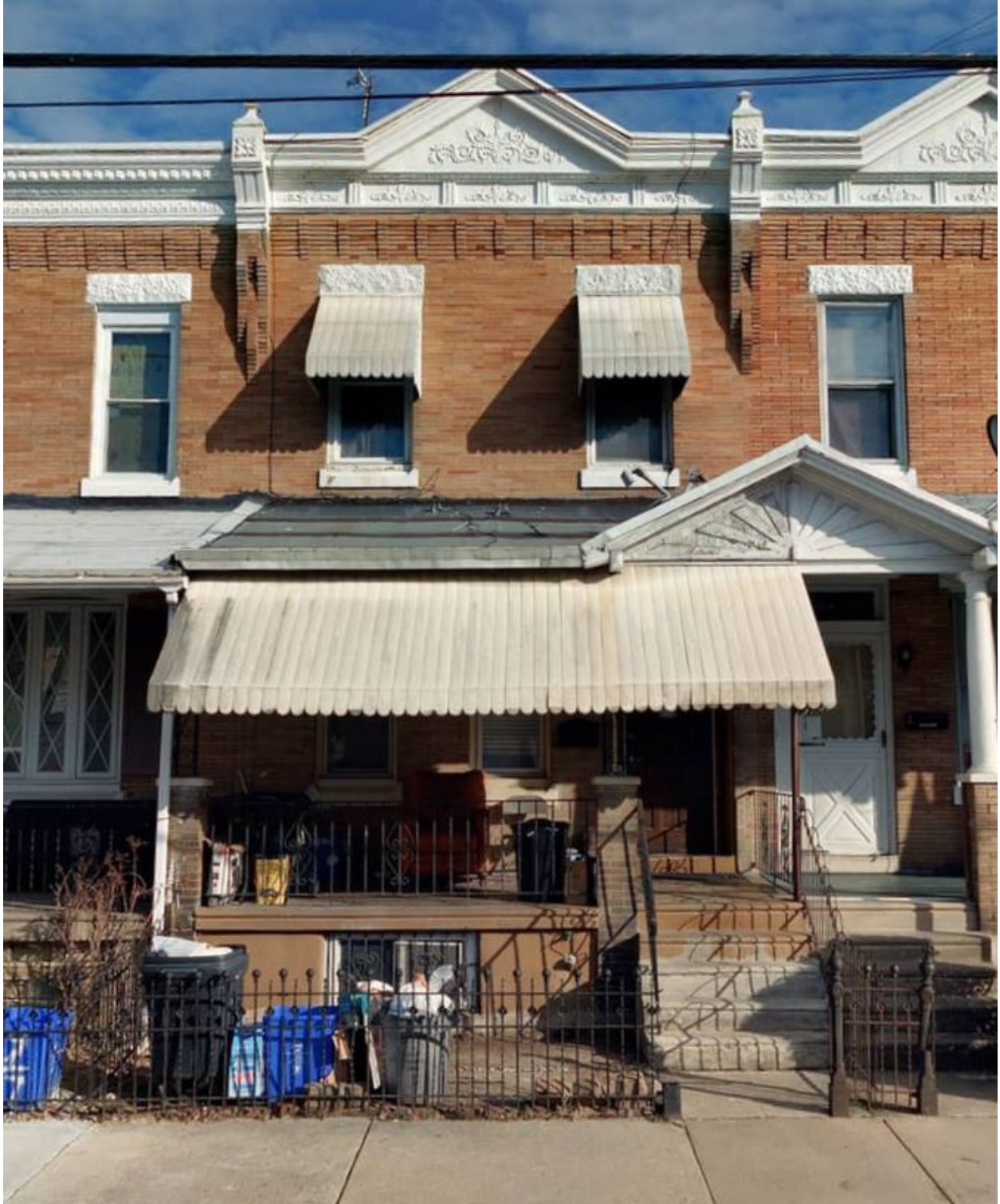
Figure 2. Front façade of 415 N. 53 rd Street, December 2022, Cyclomedia.
