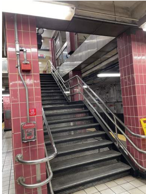
2 PLATFORM TO MEZZANINE STAIR - FINISH REPLACEMENT
