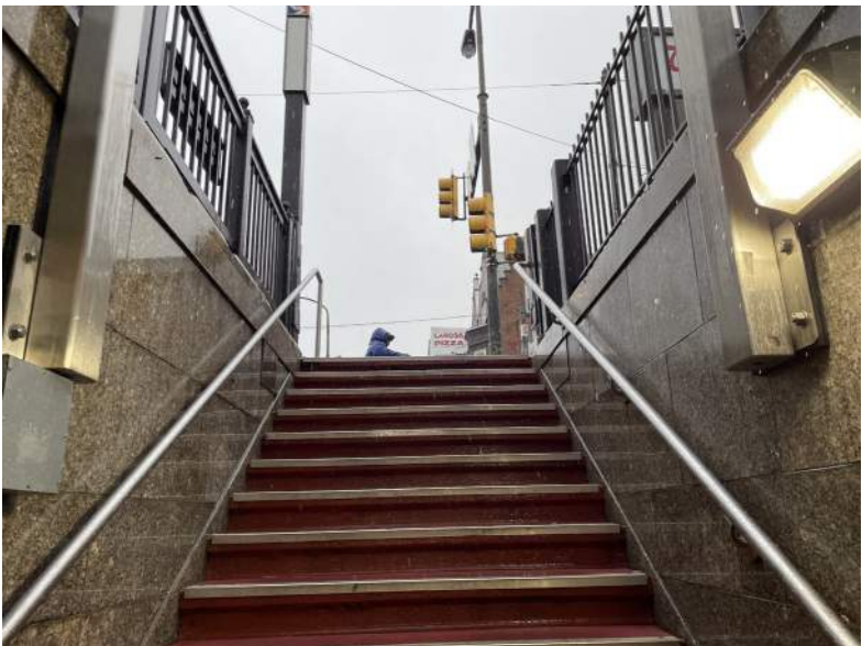
1 NORTHWEST CORNER STAIRWELL
