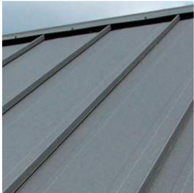
STANDING SEAM METAL ROOFING
