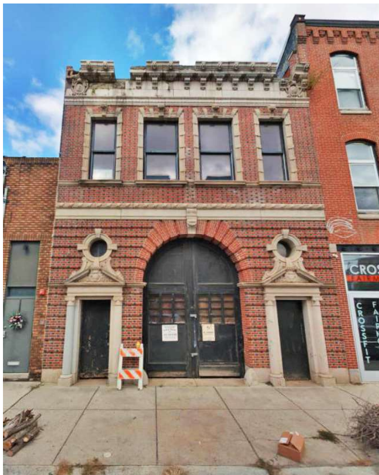
Figure 1: South elevation of the Engine 13 Firehouse, facing Parrish Street.
