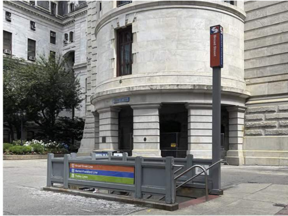
CITY HALL COURTYARD - NORTHEAST CORNER ENTRANCE STAIR
