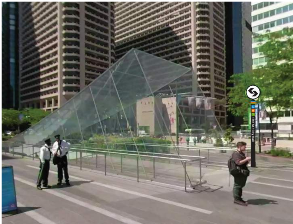
NORTHEAST STAIR (DILWORTH)
