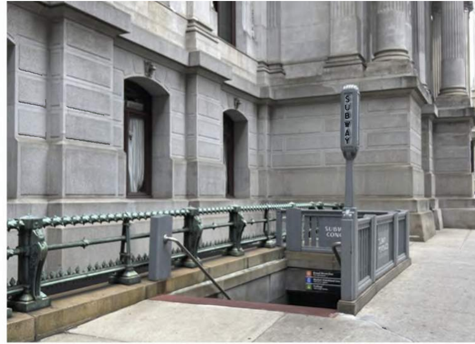
MARKET STREET & S. JUNIPER STREET - SOUTHWEST CORNER ENTRANCE STAIR
