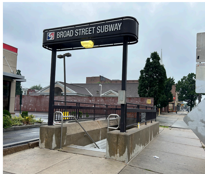
SOUTHWEST STATION ENTRANCE
