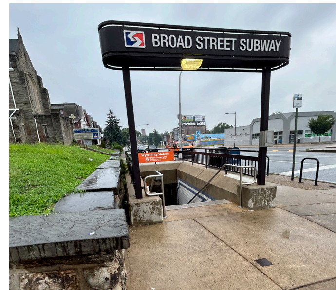
SOUTHEAST STATION ENTRANCE
