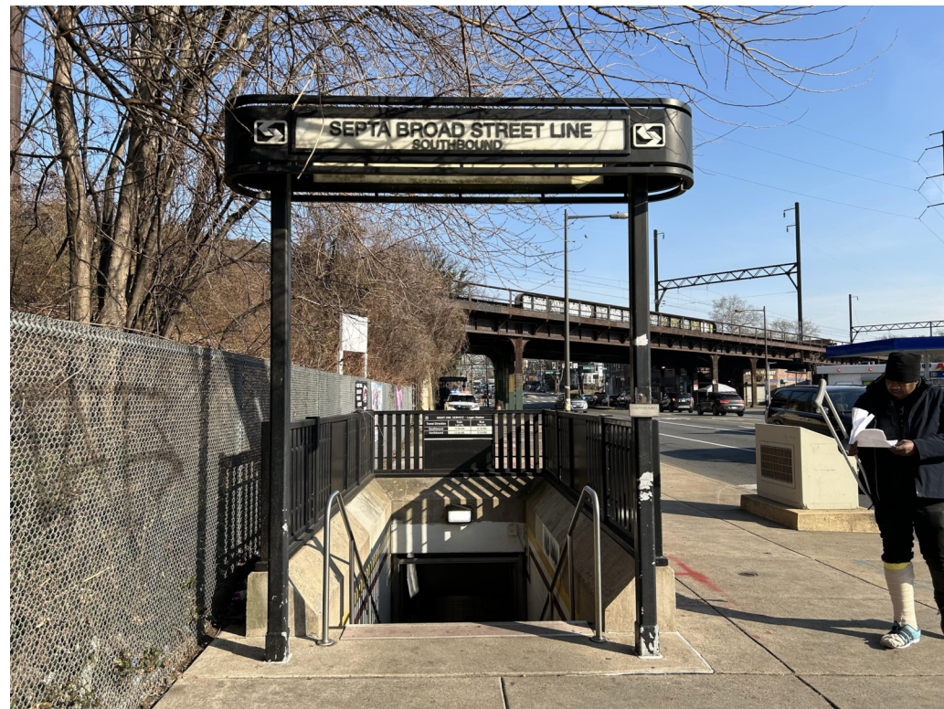
SOUTHWEST ENTRANCE (SOUTHBOUND)
