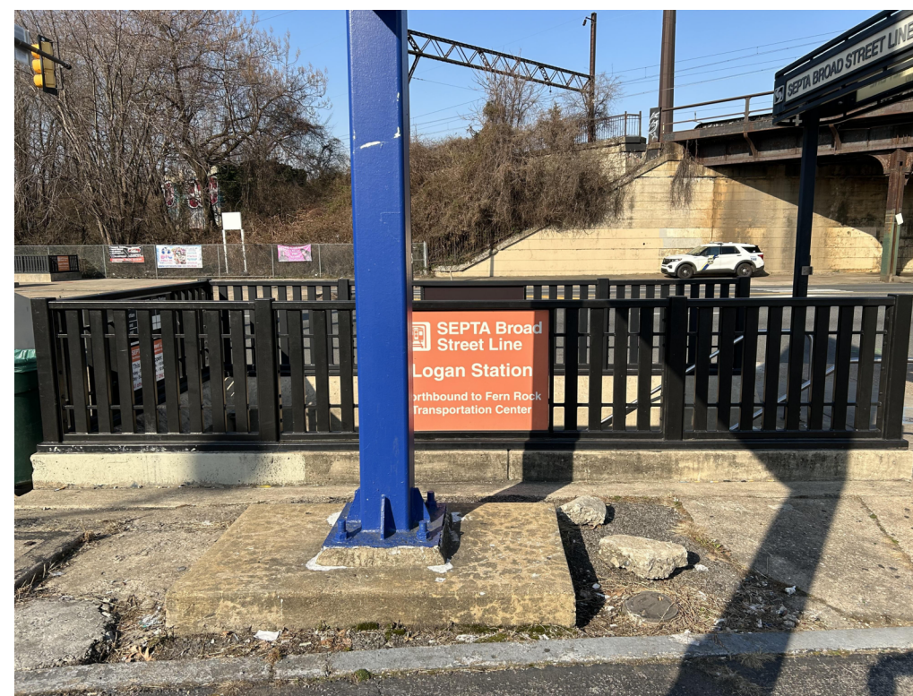
SOUTHEAST ENTRANCE (NORTHBOUND)
