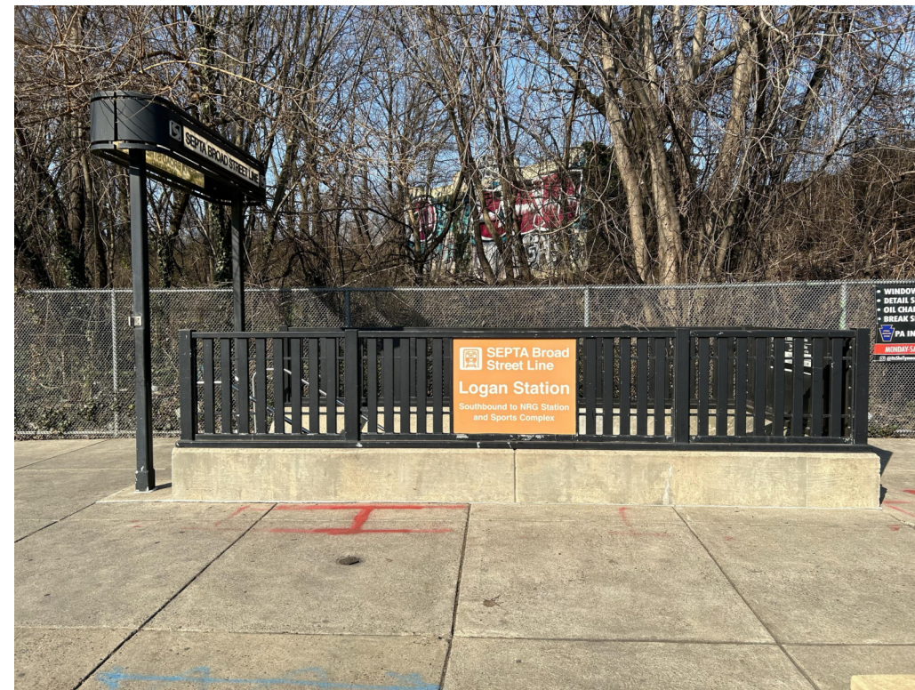
SOUTHWEST ENTRANCE (SOUTHBOUND)
