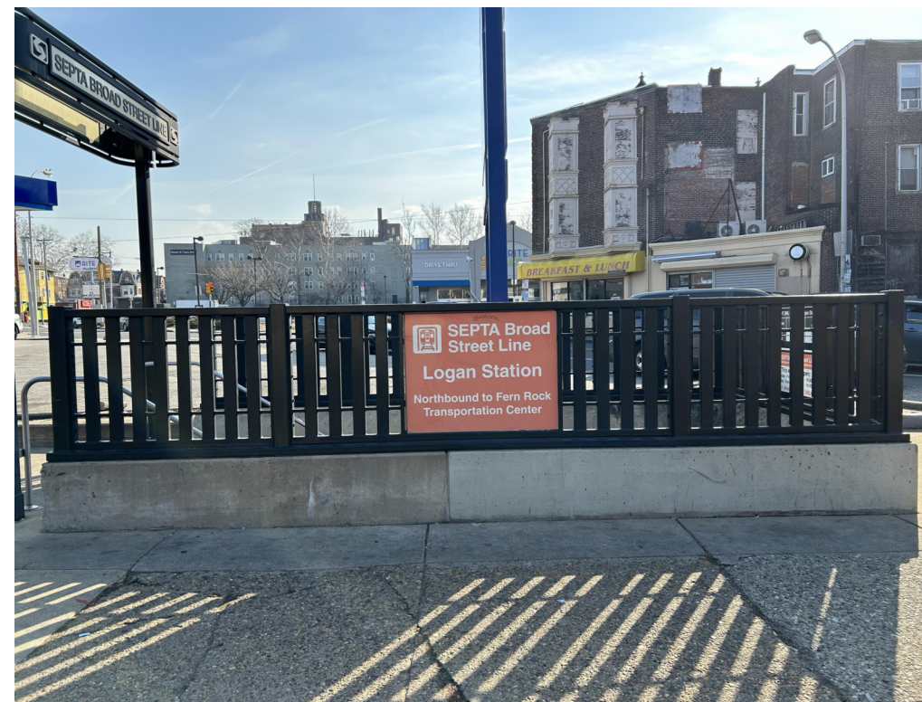
SOUTHEAST ENTRANCE (NORTHBOUND)
