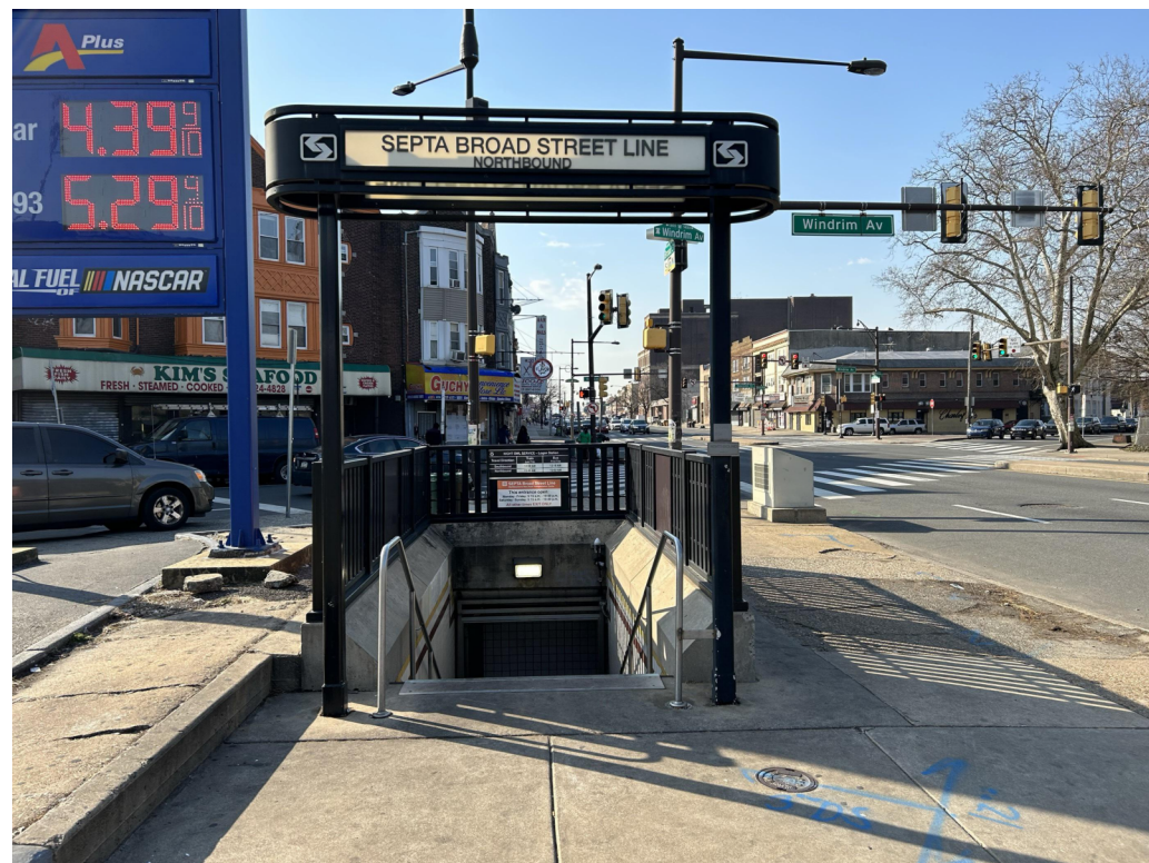
SOUTHEAST ENTRANCE (NORTHBOUND)
