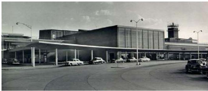
Figure 1: The new terminal at the Philadelphia International Airport, Carroll, Grisdale & Van Alen, 1947-1953 (Jacob Stelman Collection, Athenaeum of Philadelphia).
