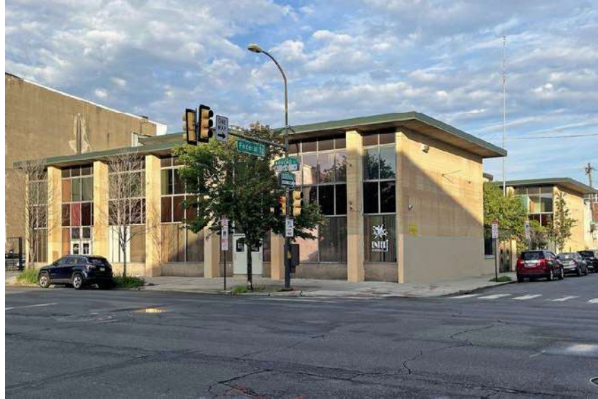
Photo 2: East and north elevations, looking southwest (July 2023).
