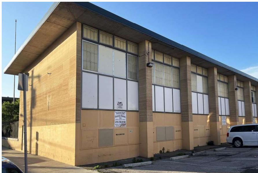
Photo 5: North and west elevations, looking southeast from Federal Street (July 2023).
