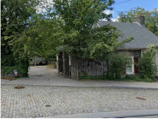
① EXISTING ENTRY CARRIAGE HOUSE
