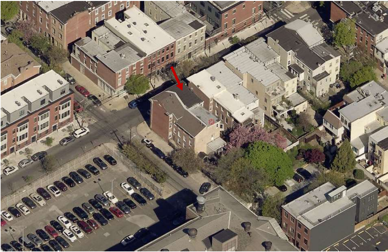
Figure 5: Aerial view of 627 N 16 th St from the Southeast:
