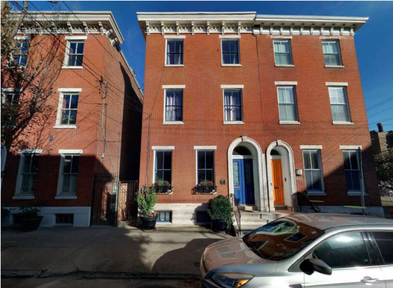
Figure 2: View of front façade of 627 N 16 th St from N 16 th St:
