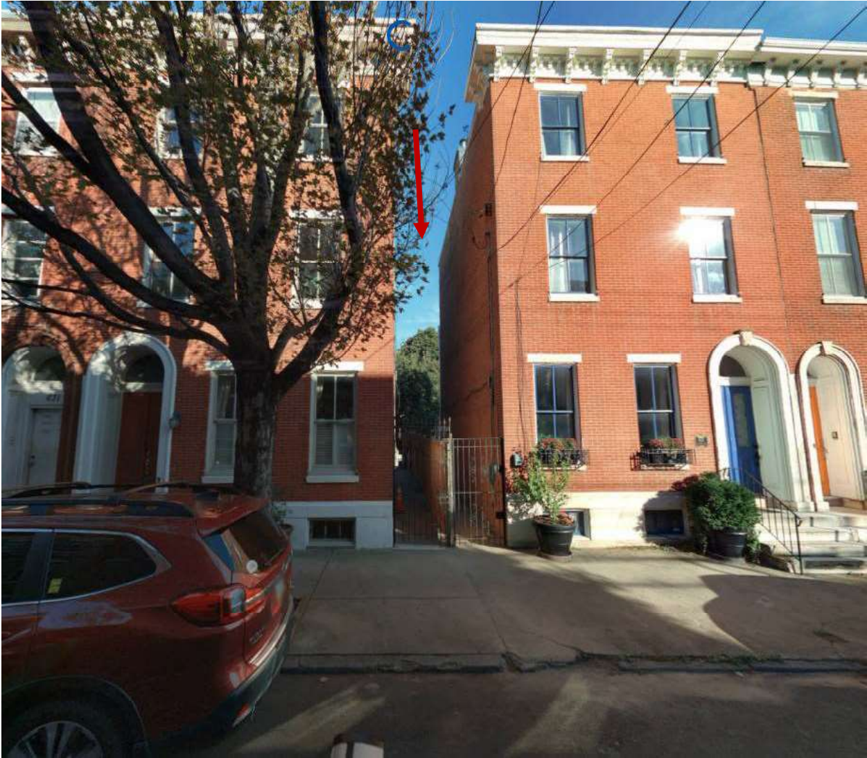
Figure 3: View down side of 627 N 16 th St from N 16 th St, arrow indicates where addition will go:
