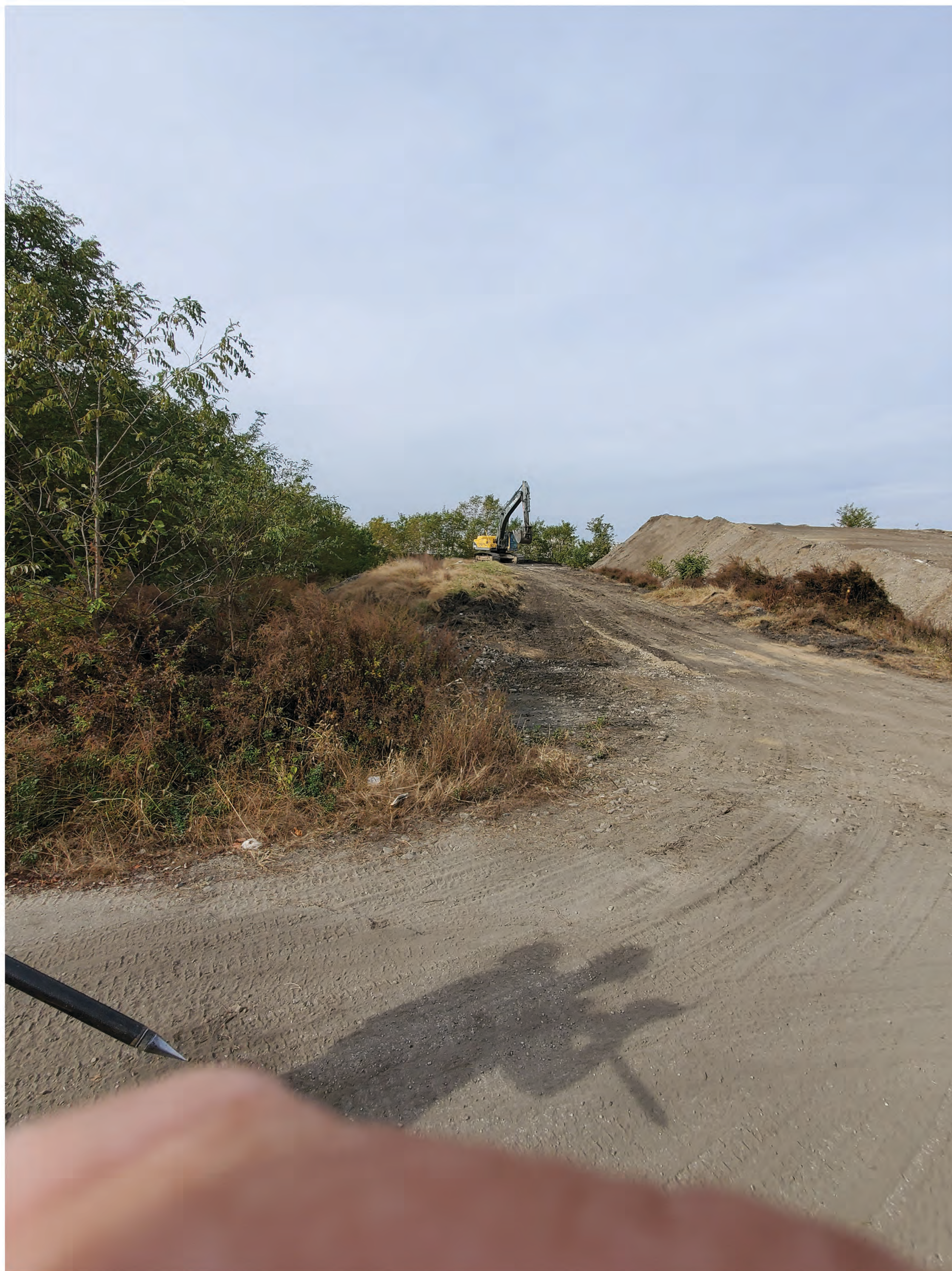
Photo 3 - View from Site Road Facing West
