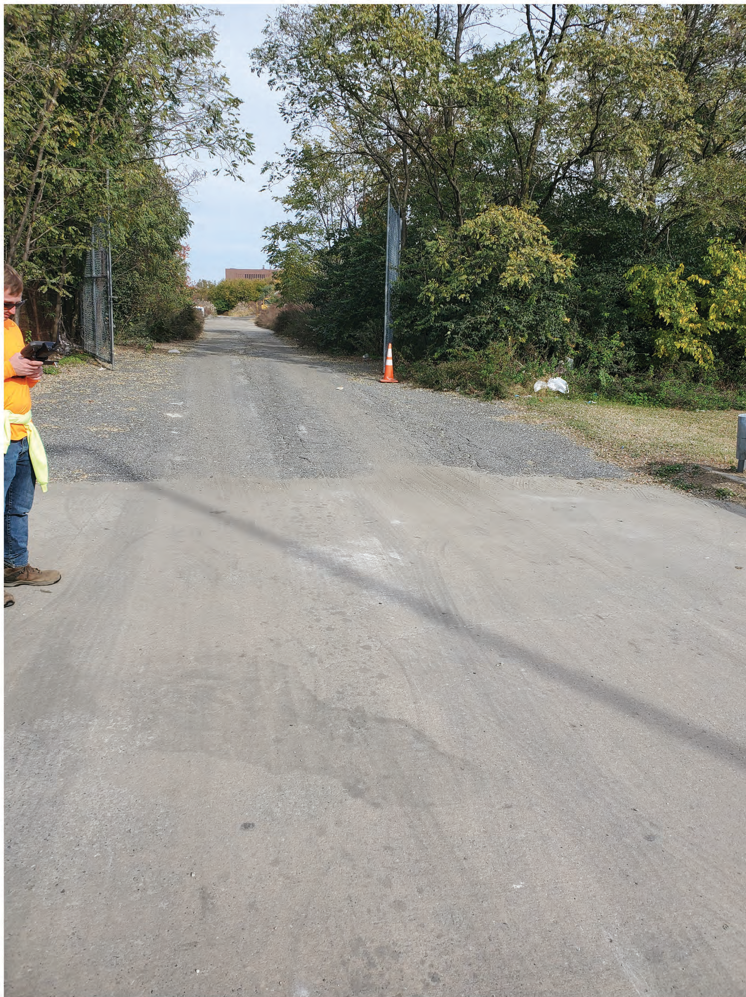
Photo 1 - View of Site from Escort Street Facing North
