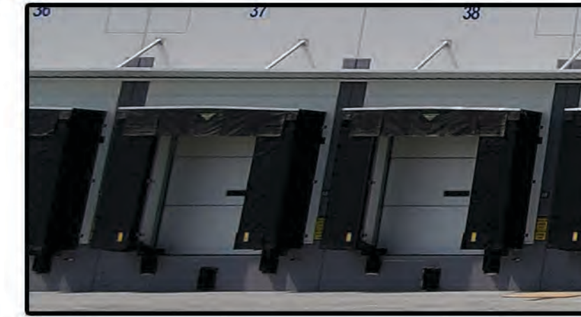
#3 INSULATED OVERHEAD DOORS WITH DOCK SHELTERS
