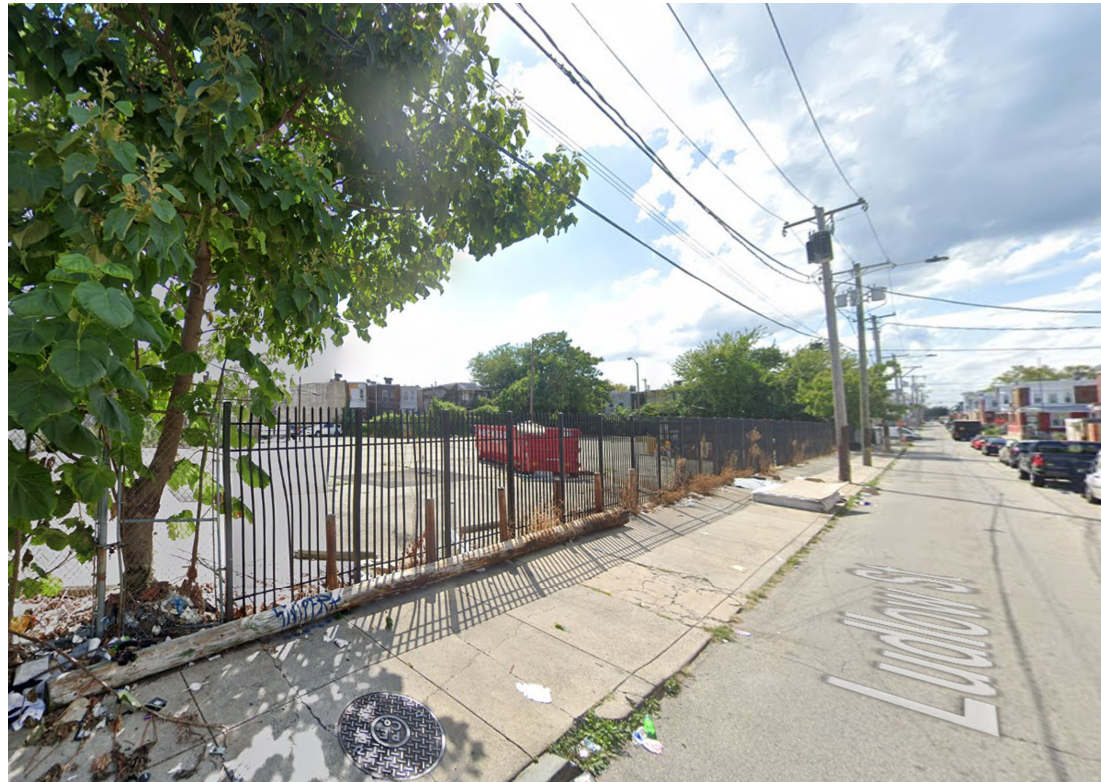
Photo 7 – Ludlow Street property frontage
