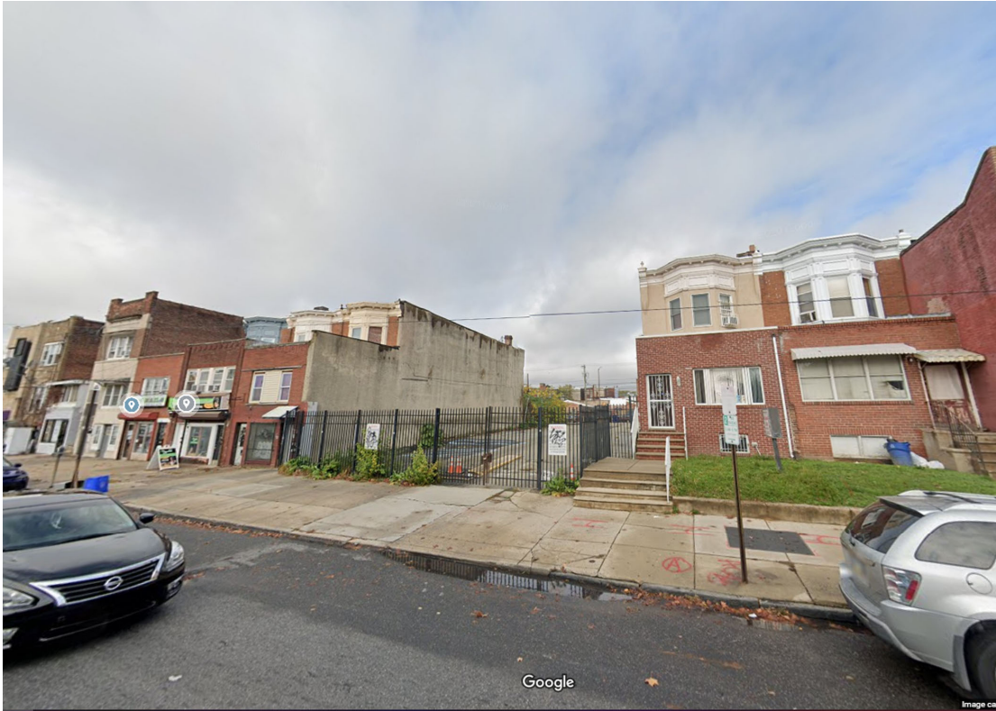
Photo 2 – Looking at Chestnut street property frontage
