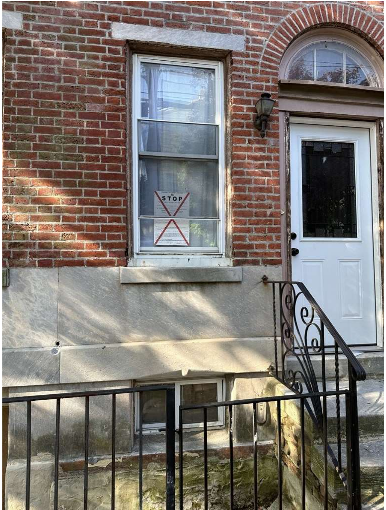
Figure 6. 242 Christian Street, showing new entry door. May 2024.
