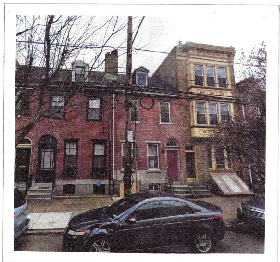
PHOTO - 1 PREMISE FRONT
