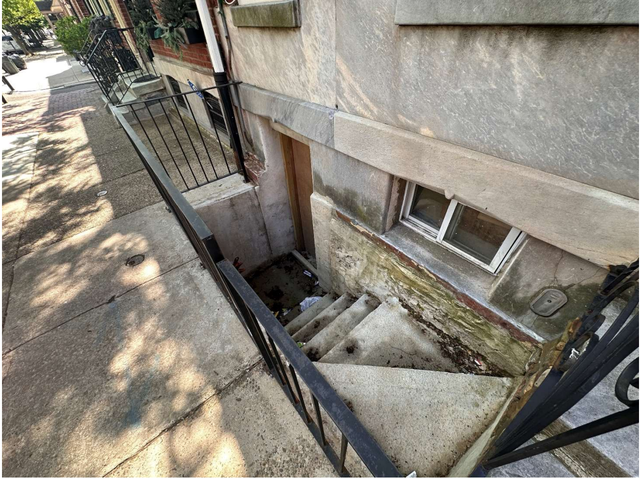
Figure 8. 242 Christian Street, showing basement entrance. May 2024.
