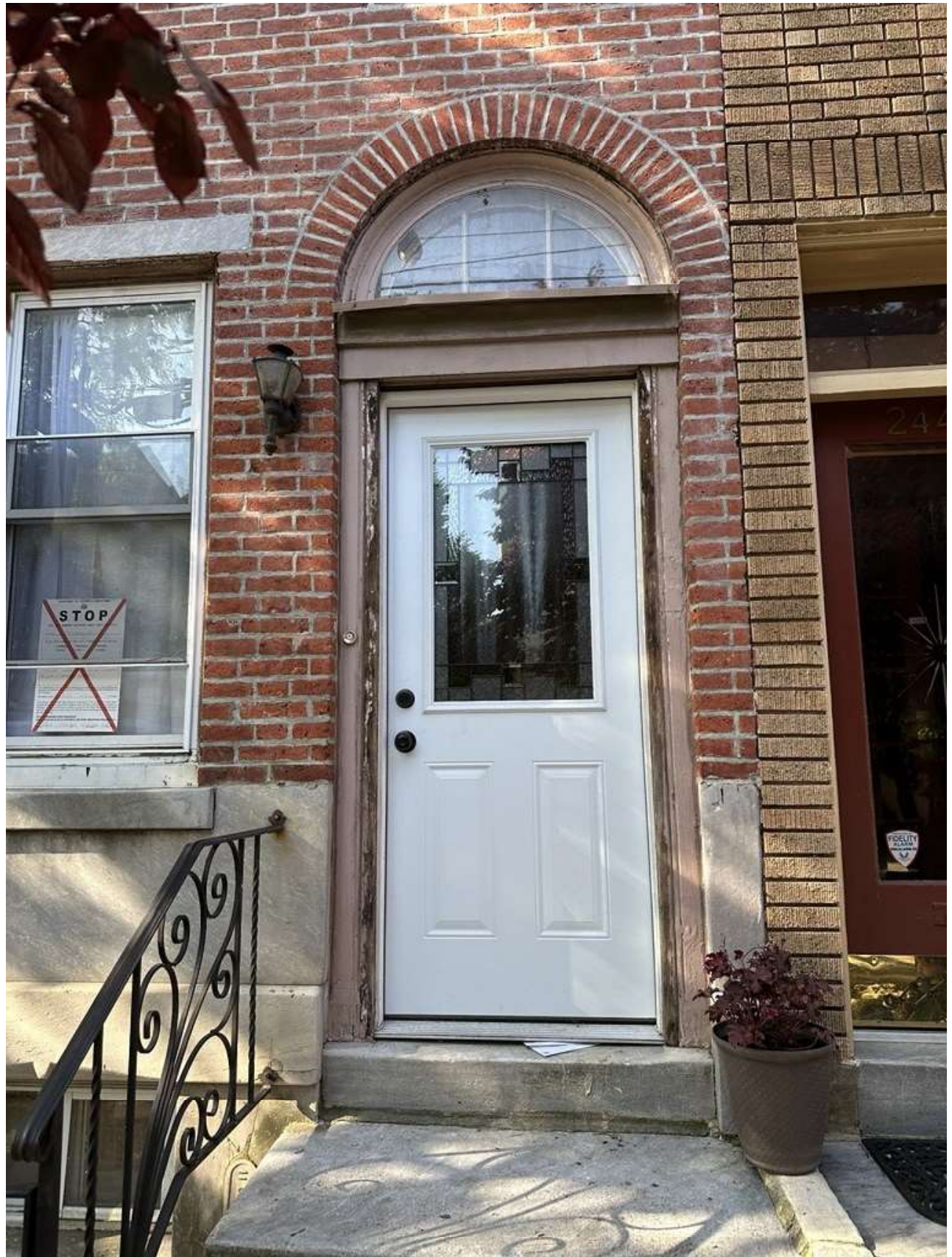
Figure 5. 242 Christian Street, showing new entry door. May 2024.
