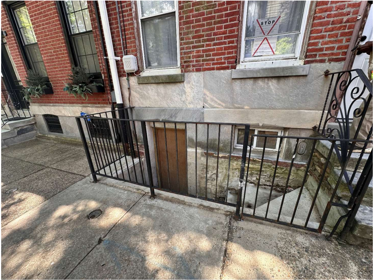
Figure 7. 242 Christian Street, showing basement entrance. May 2024.
