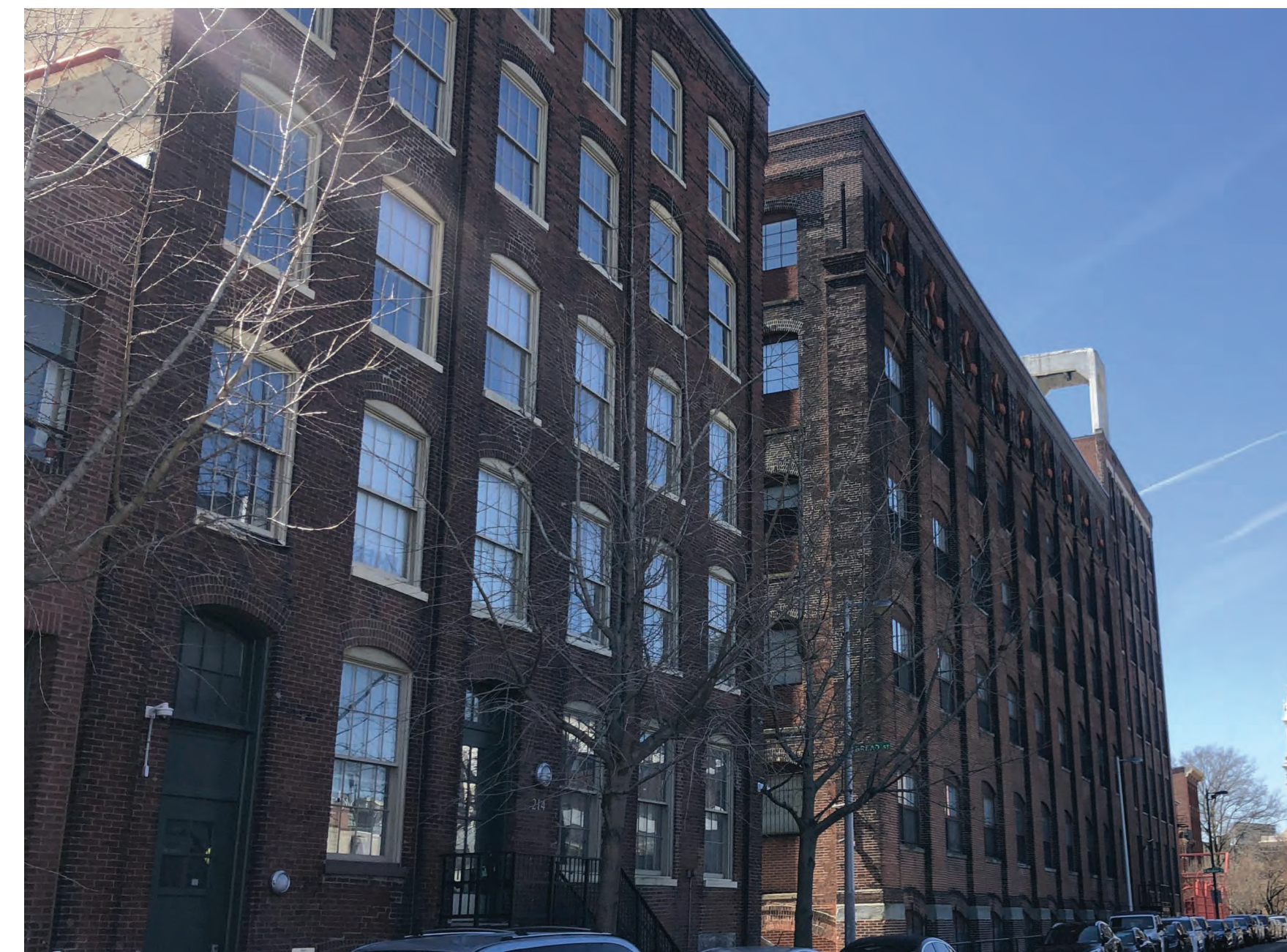
6 VIEW OF 214-18 NEW STREET
