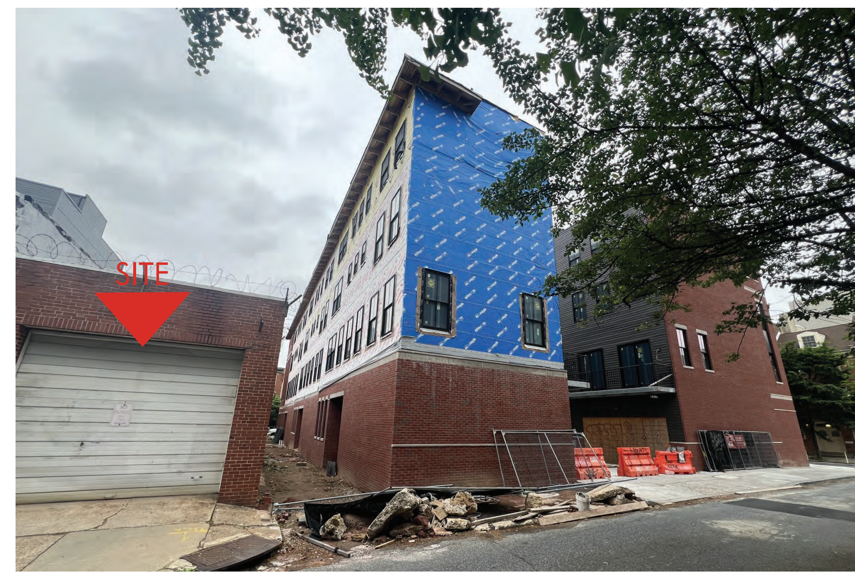
3 REAR VIEW OF 244-58 N. 2ND STREET
