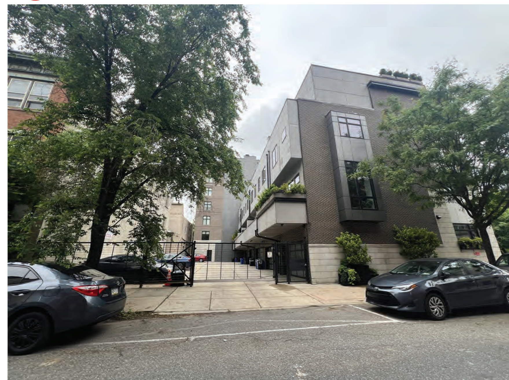
8 REAR VIEW OF 300-10 N. 2ND STREET
