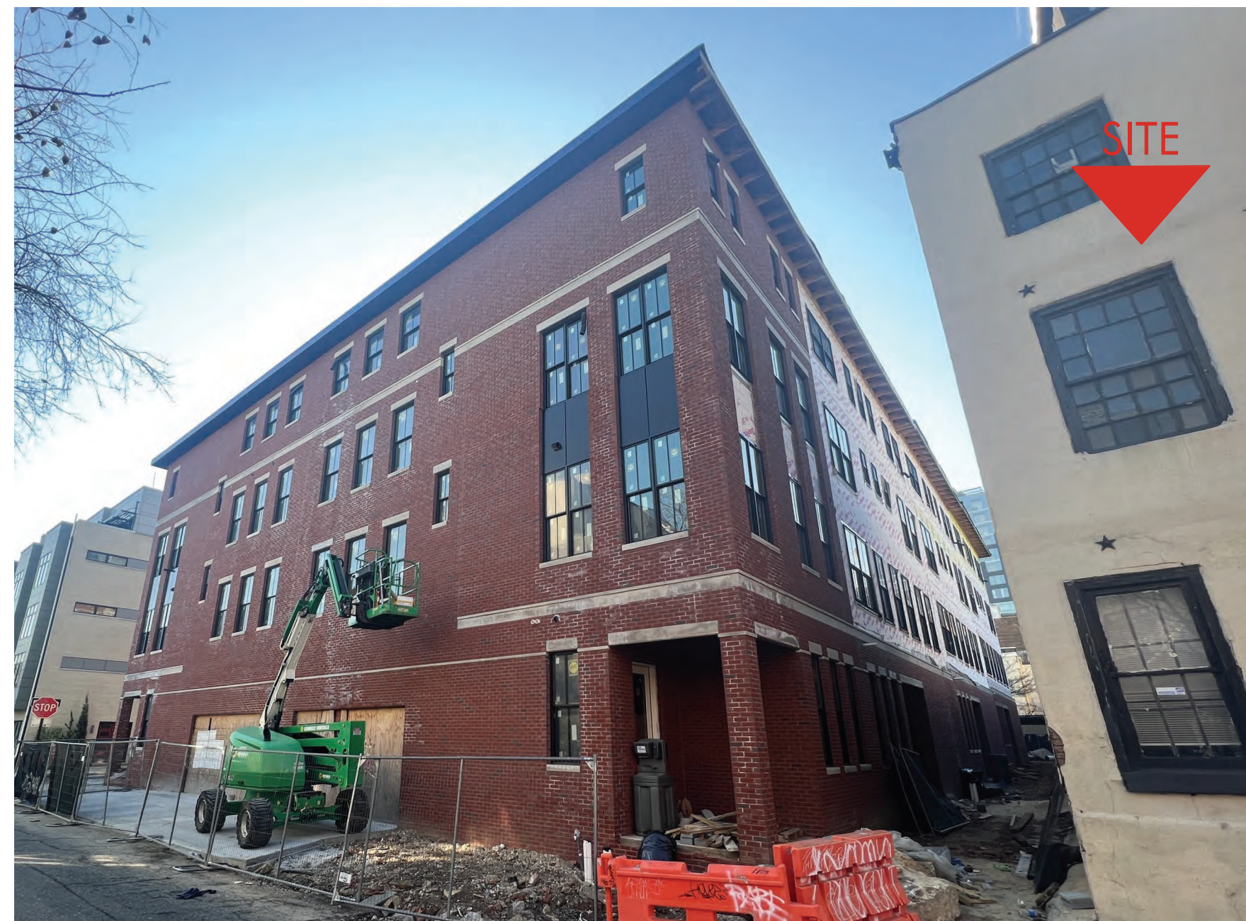
4 FRONT VIEW OF 244-58 N. 2ND STREET
