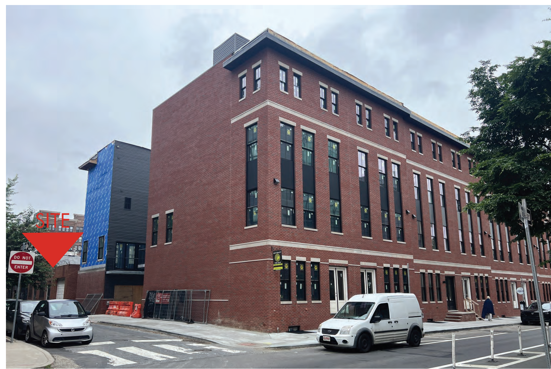
1 FRONT VIEW OF 244-58 N. 2ND STREET
