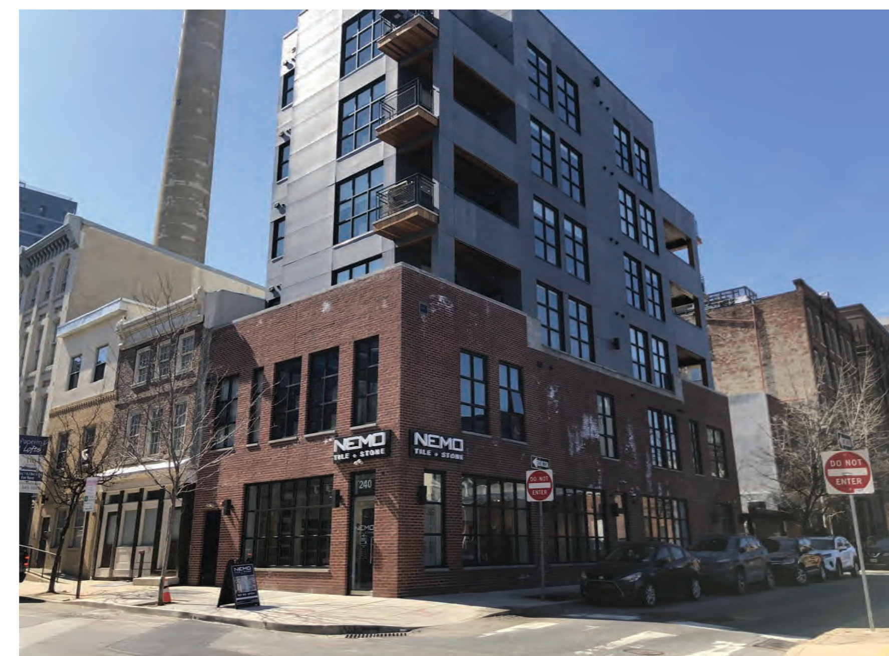
14 FRONT/SIDE VIEW OF 240-42 N. 2ND ST
