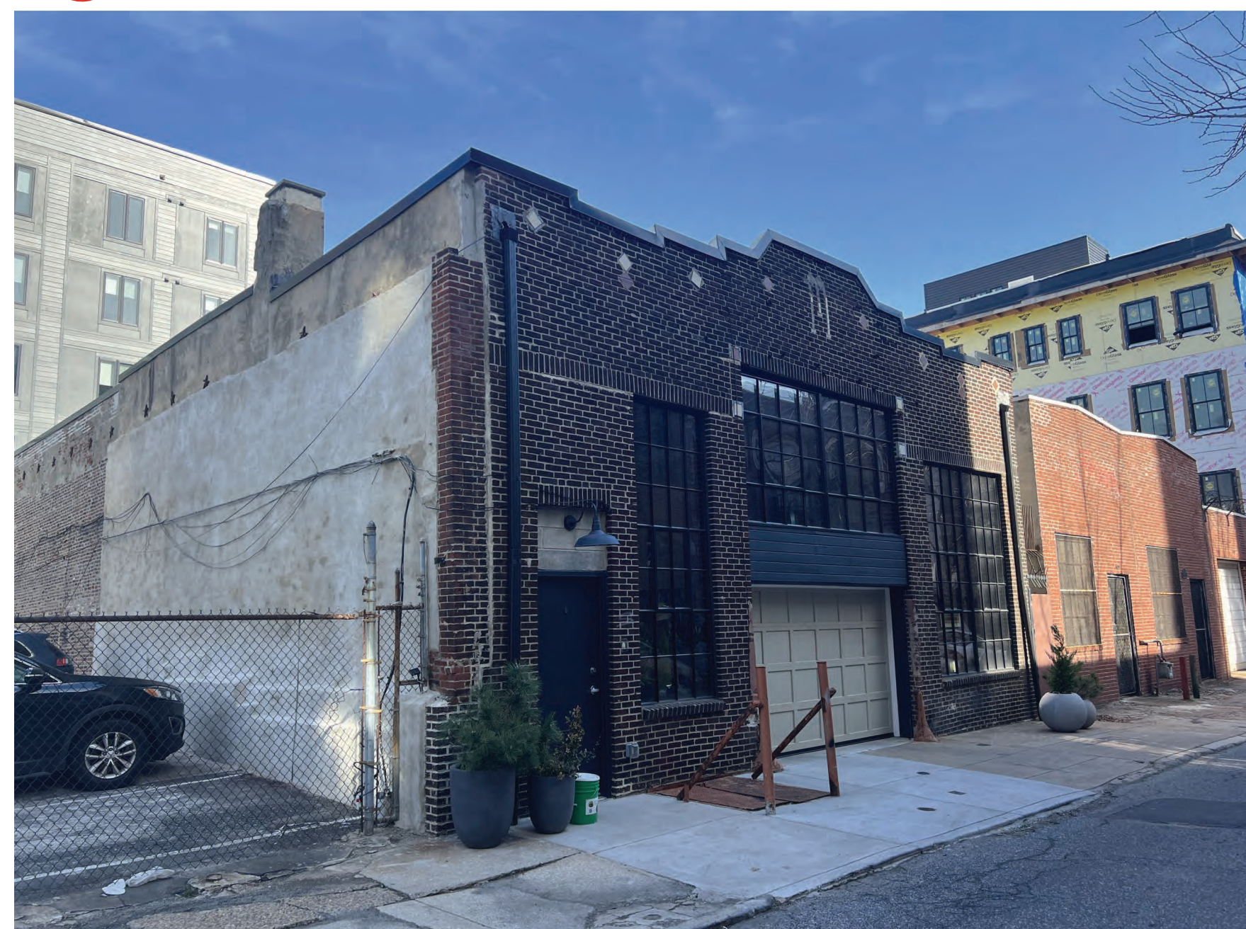
7 FRONT VIEW OF 213-15 NEW STREET
