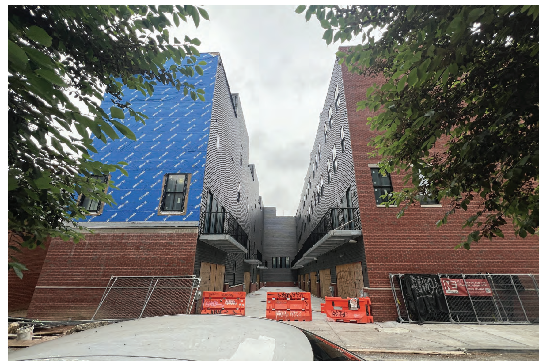
2 REAR VIEW OF 244-58 N. 2ND STREET
