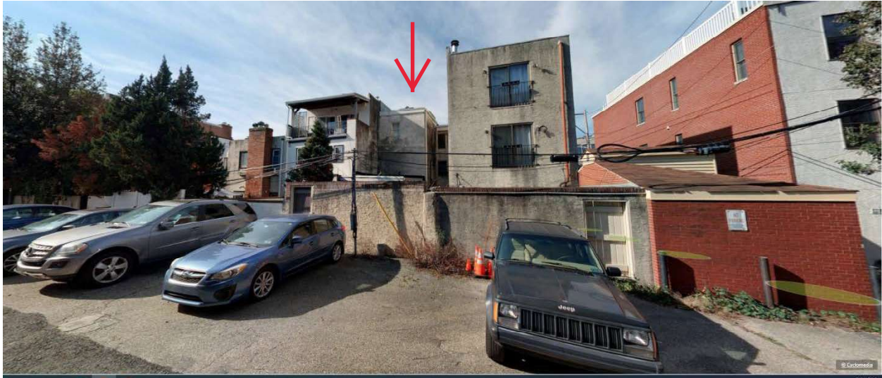
Figure 3. West Side 600 Block S. Hoard Street, 2021. Source: Cyclomedia.phila.gov
