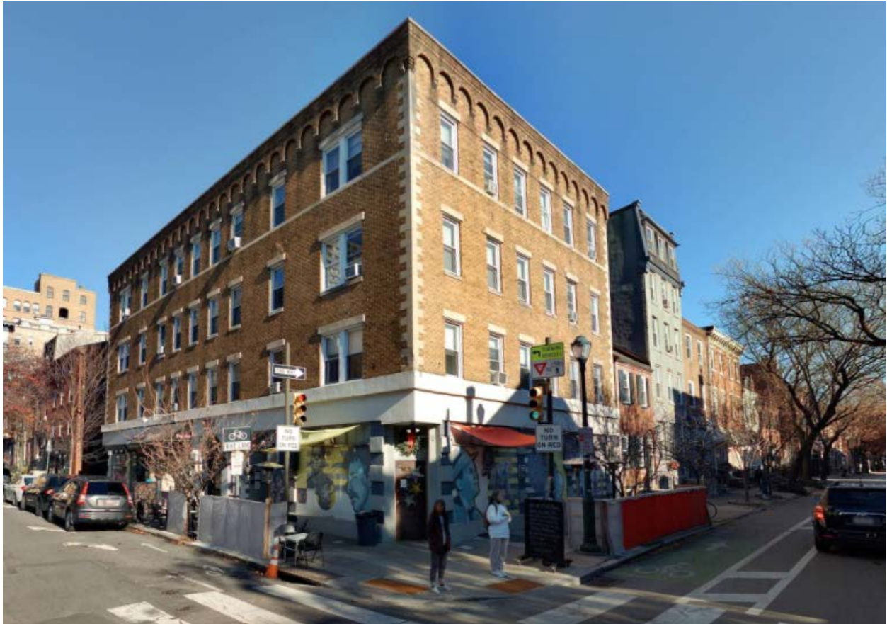
Photograph 20: Looking northeast from the intersection of 13 th and Pine Street. Cyclomedia, December 2021.
