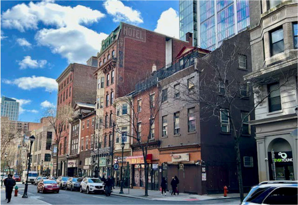
Photograph 2: Looking southeast along the 1200 block of Walnut Street.
