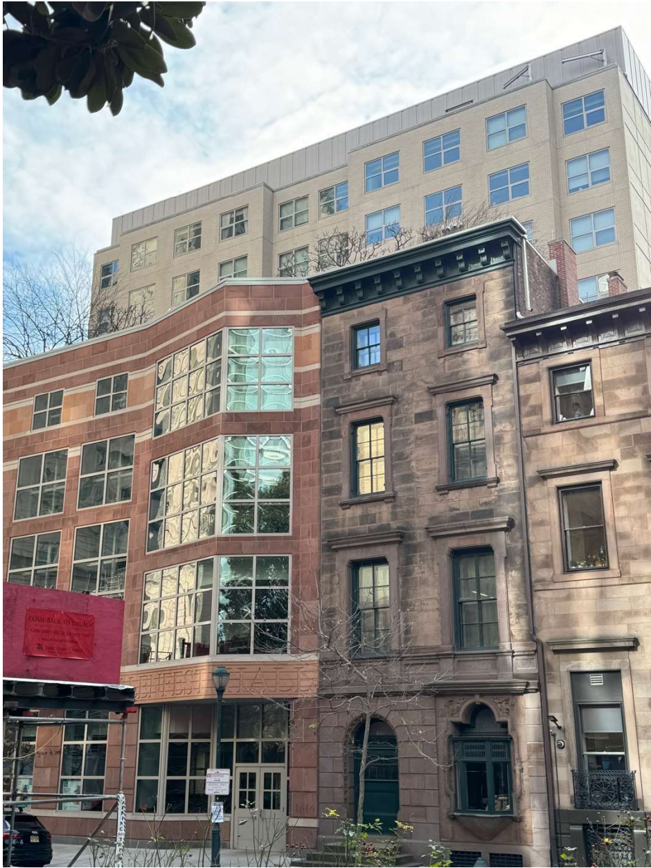
1610-1618 Locust St-8 stories building
