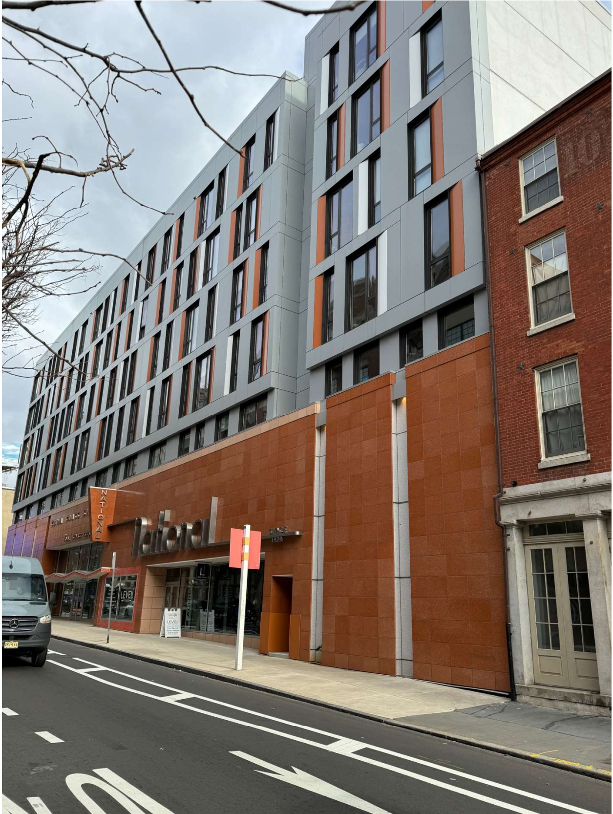
109 N 2nd St-7 stories building.
