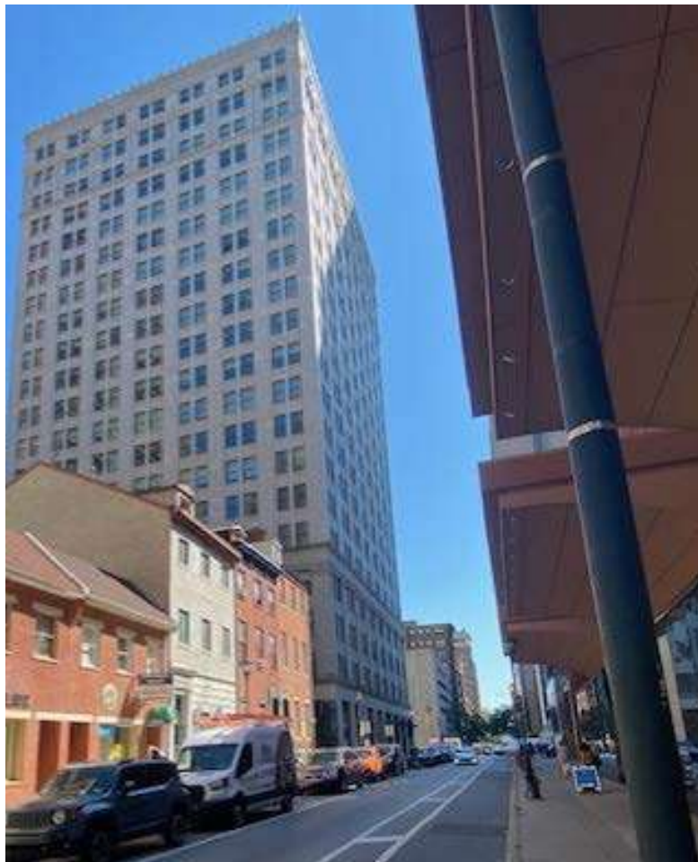
Figure 3. Spruce Street east of proposed building.
