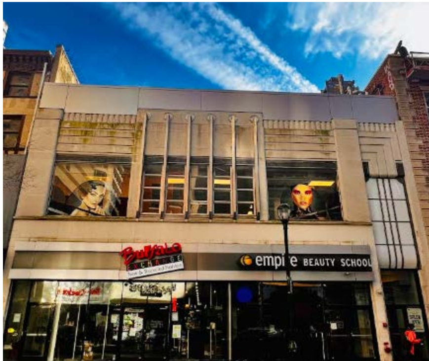
Figure 1: The primary (north) elevation of the subject property. Source: Oscar Beisert, 2022.
