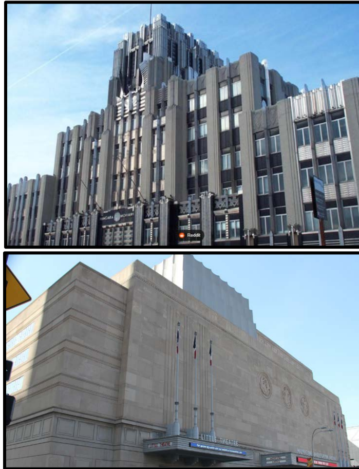
Figure 15. Top: The Niagara Mohawk Power Corporation in Syracuse, New York. Source: Reddit. Figure 16. Bottom: Kansas City Municipal Auditorium, Kansas City, Missouri. Source: Living New Deal.
