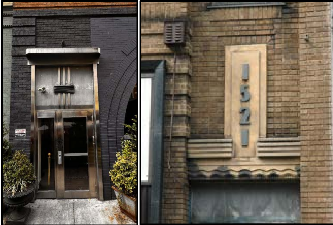
Figure 8. Left: The pedestrian entrance of the rear (south) elevation. Source: Oscar Beisert, 2022. Figure 8.5. Right: The rear address in the Art Deco style. Source: Oscar Beisert, 2022.
