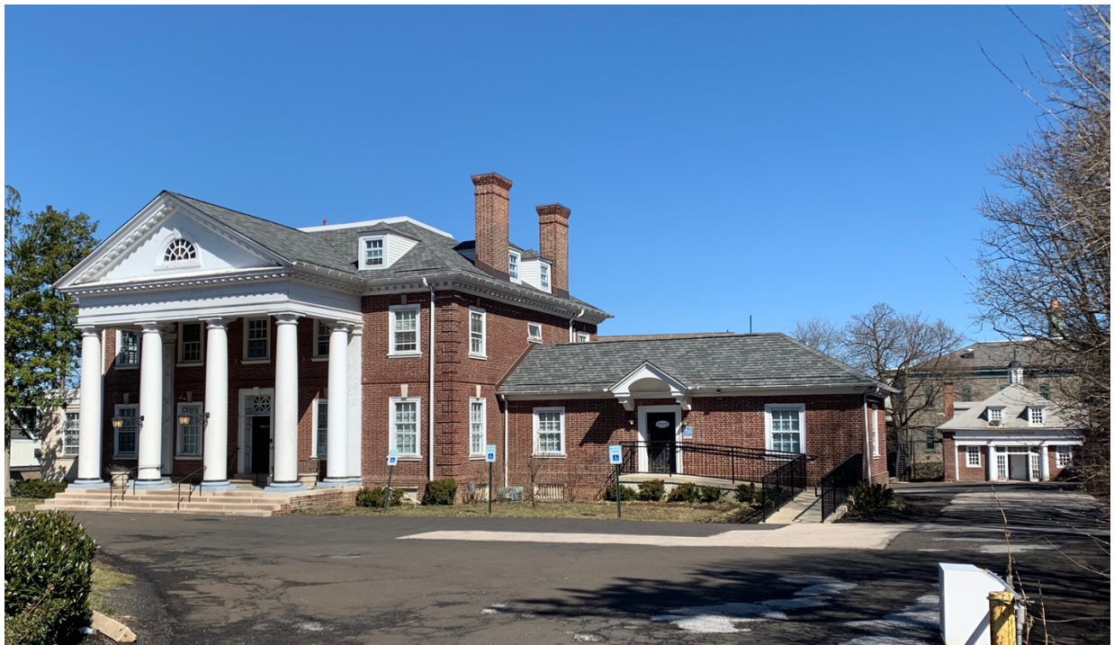
Figure 1: Front (southwest) elevation as viewed from Germantown Avenue.
