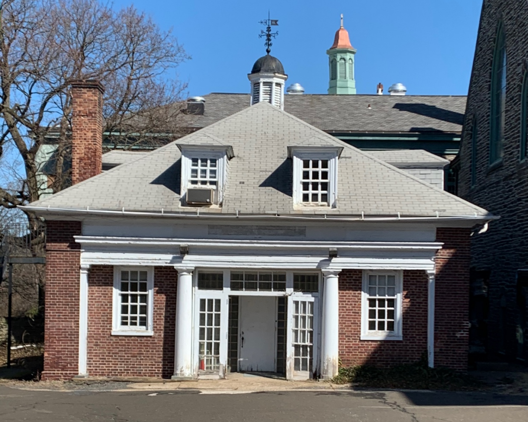
Figure 5: Carriage house, southwest (front) elevation.
