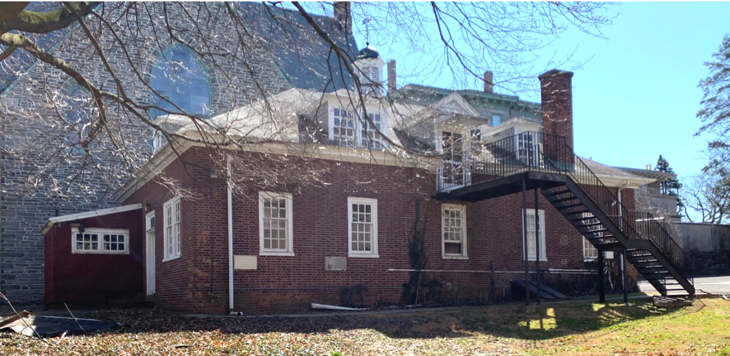
Figure 6: Carriage house, northwest (side) elevation
