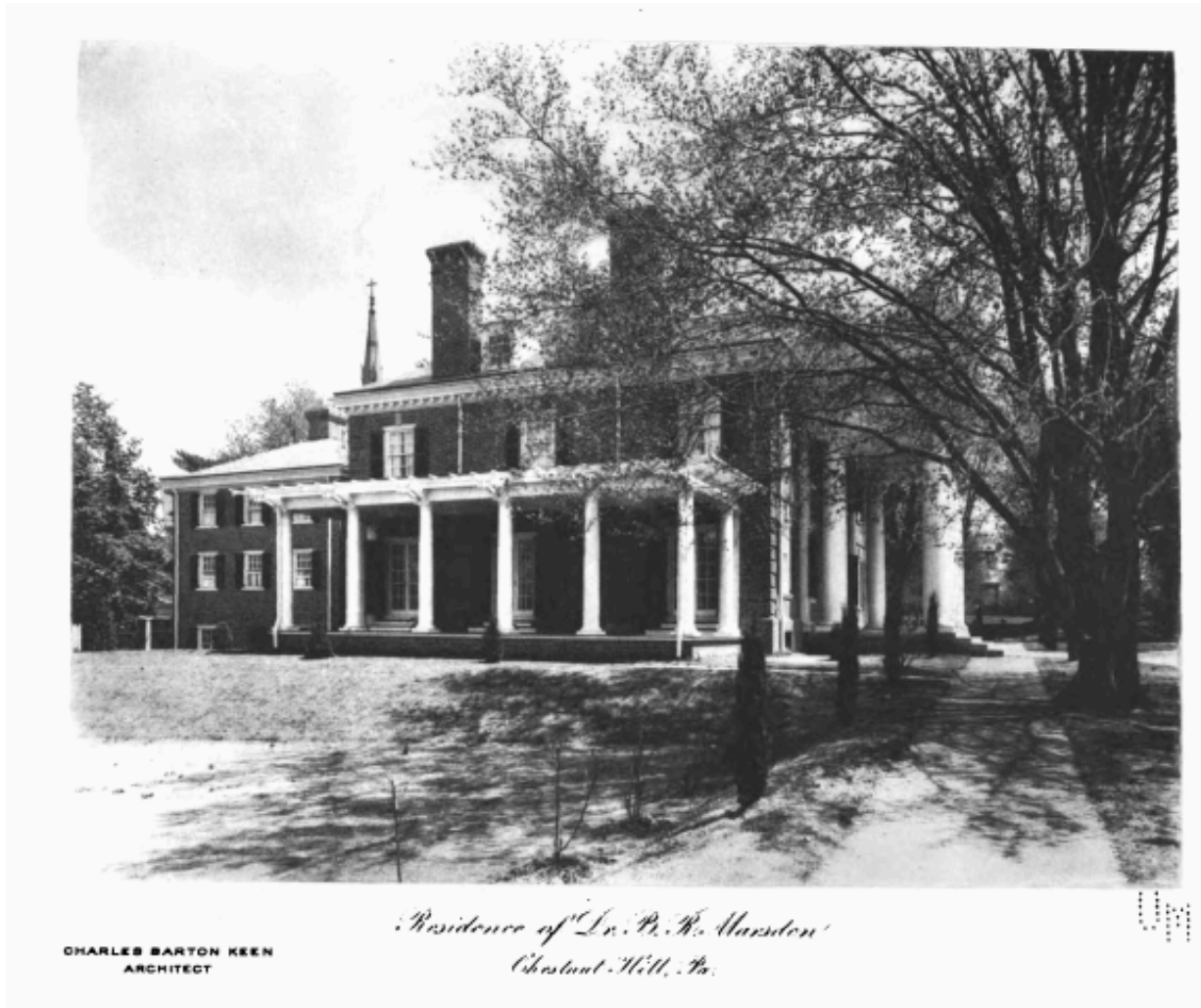
Figure 14: New York Architect , Vol. 3, no. 5, May 1909. Side view of northwest elevation with original pergola replaced by 1912 addition.
