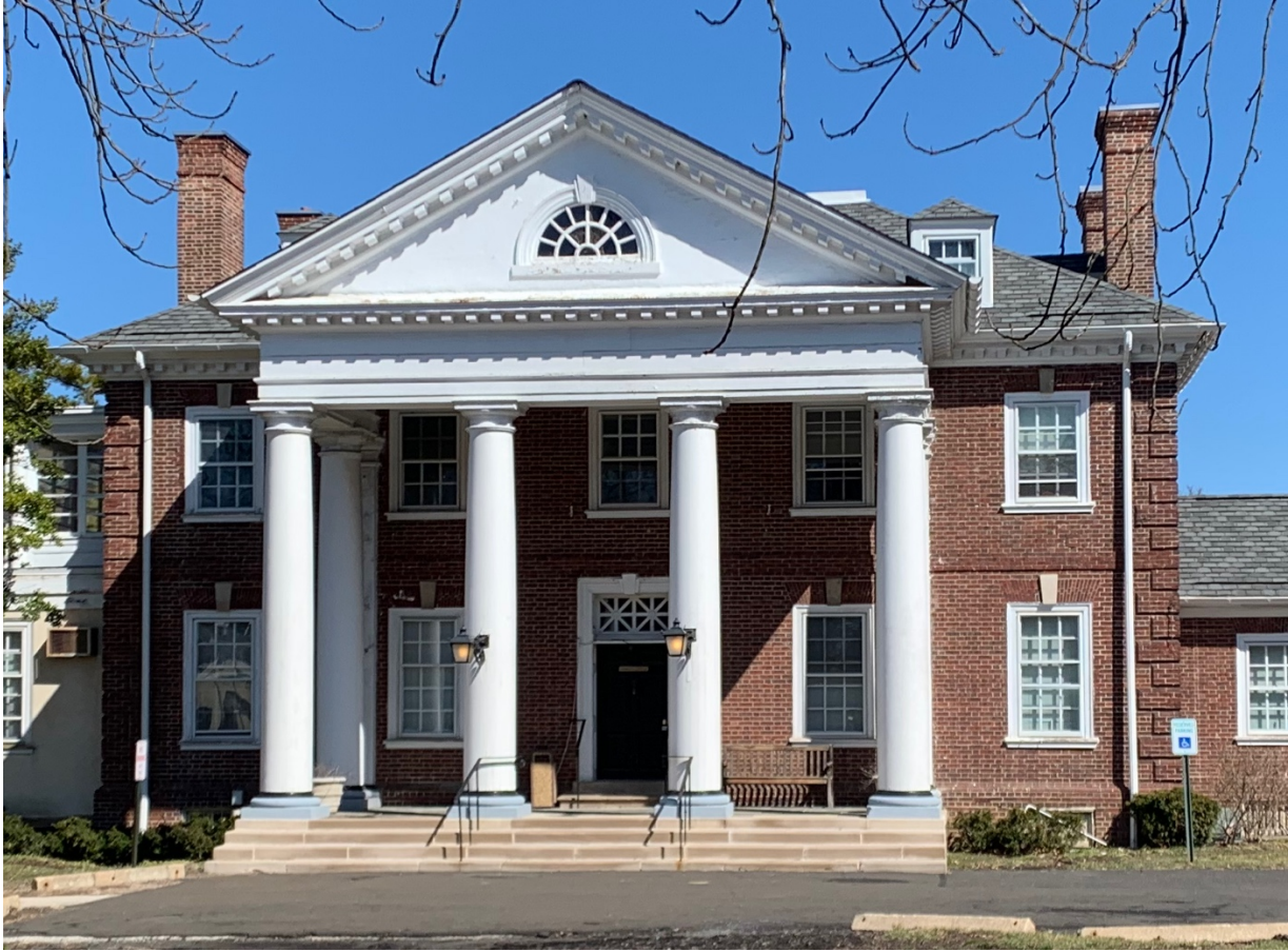
Figure 2: Southwest elevation detail
