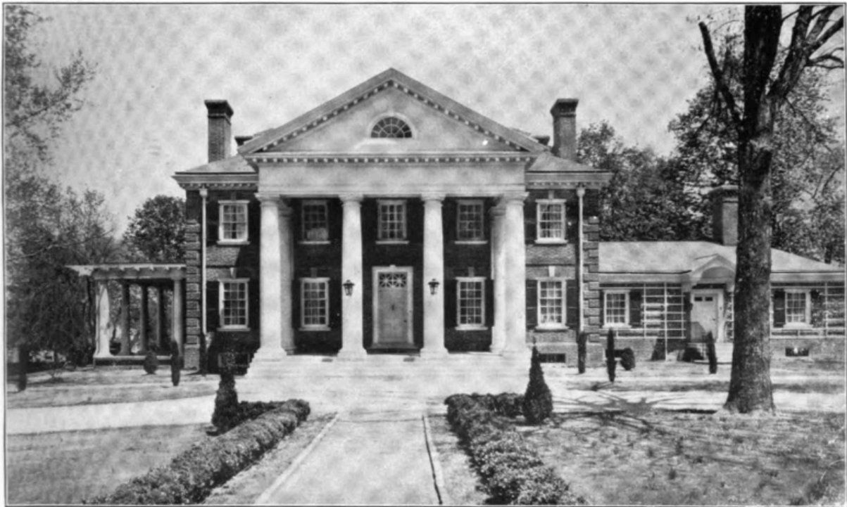
STREET FAÇADE, DR. MARSDEN'S HOUSE, CHESTNUT HILL, PHILADELPHIA CHARLES BARTON KEEN Architect
