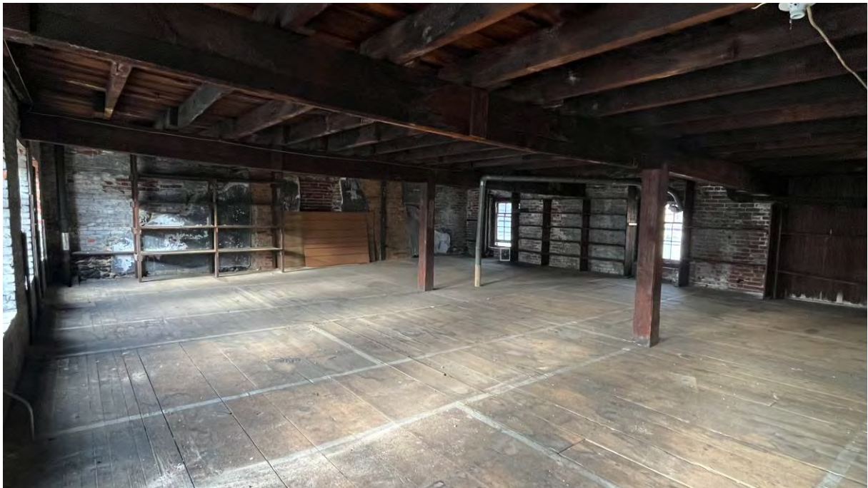
Third floor of office space – low ceilings
