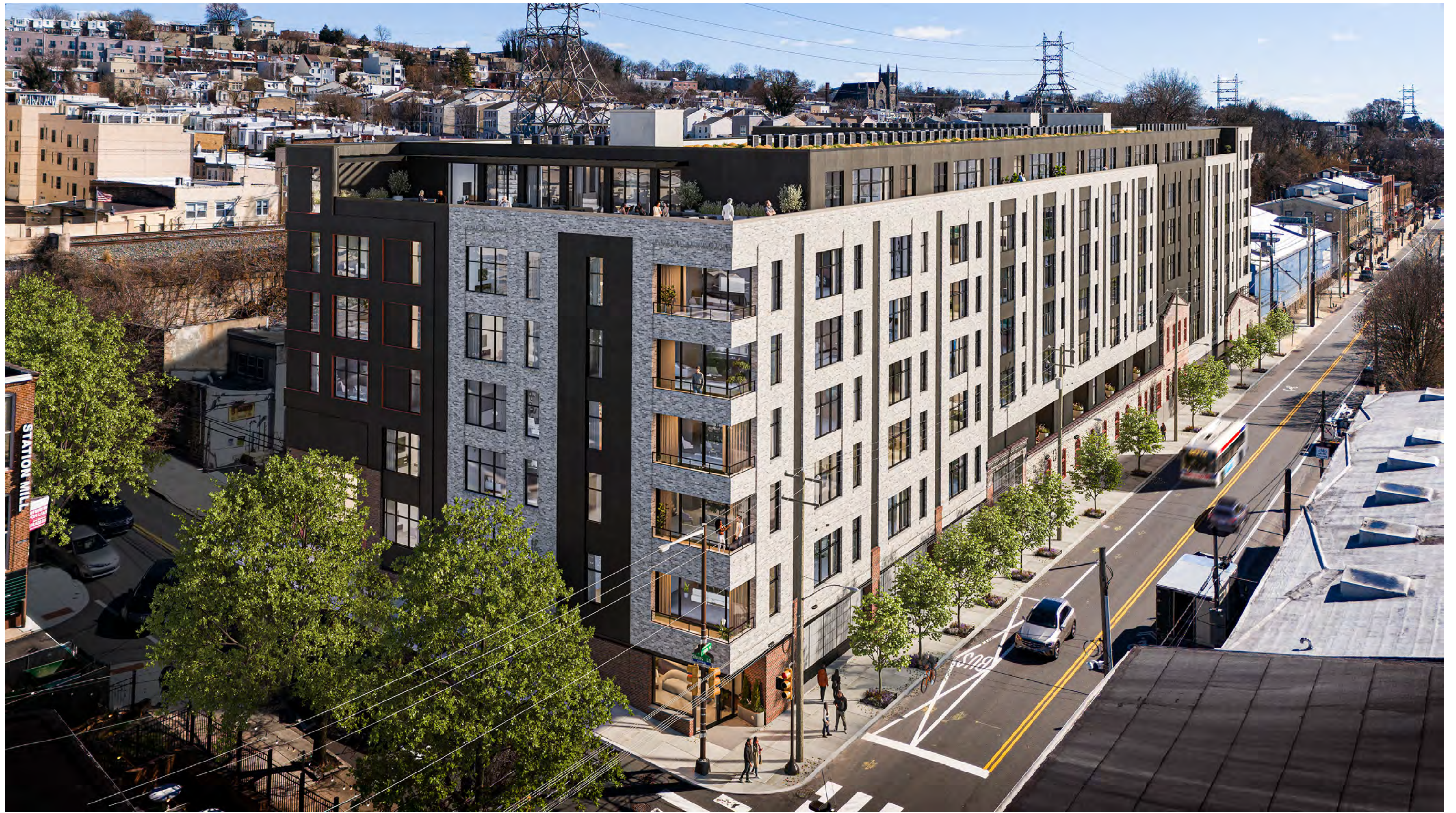
Aerial View looking Southeast
