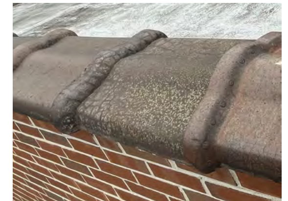
16 Existing Terracota Coping
