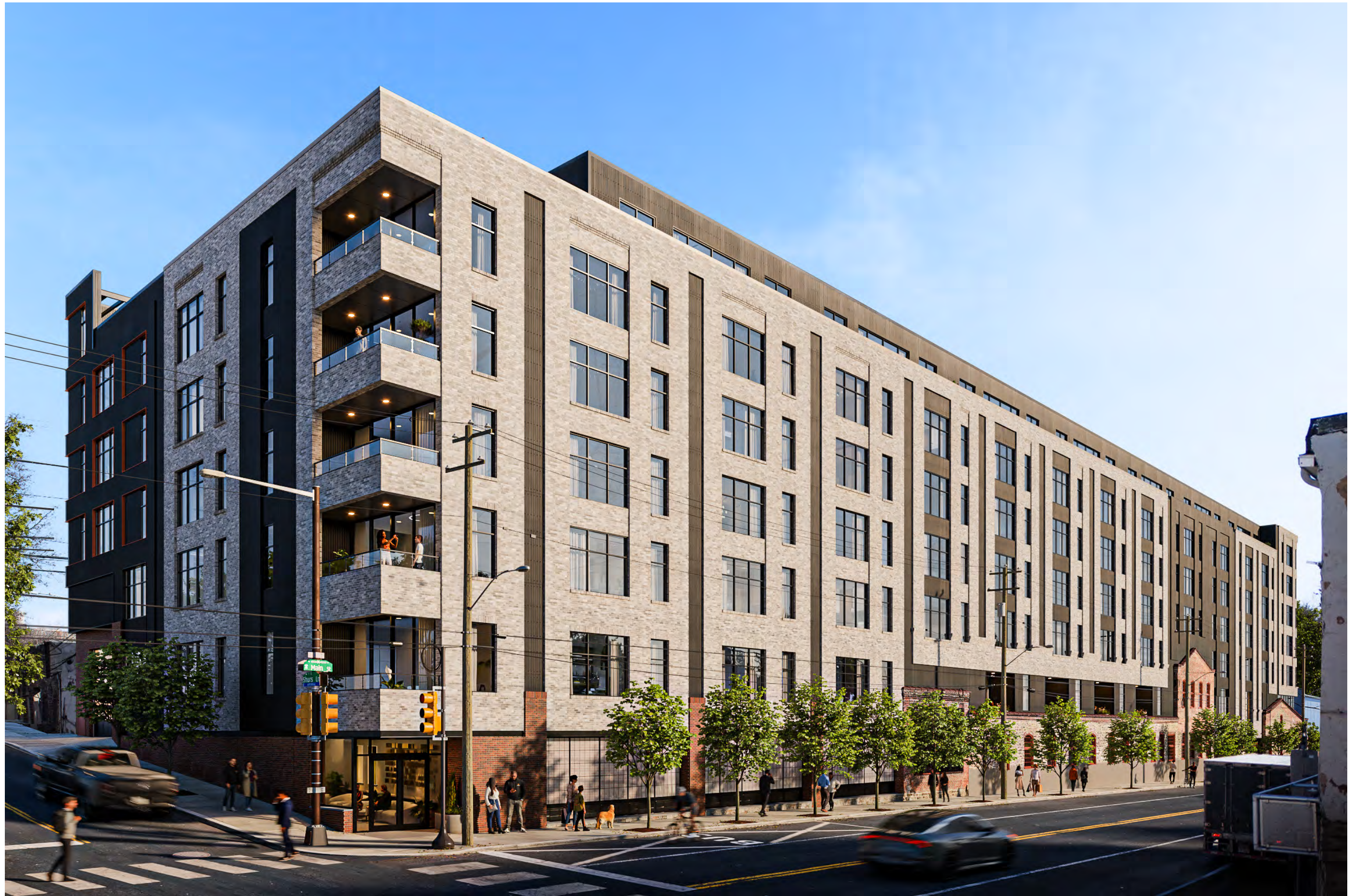
View looking East on Main Street & South on Shurs Lane
