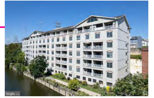
Watermill at Manayunk 2 Leverington Avenue, Philadelphia 7 Stories
