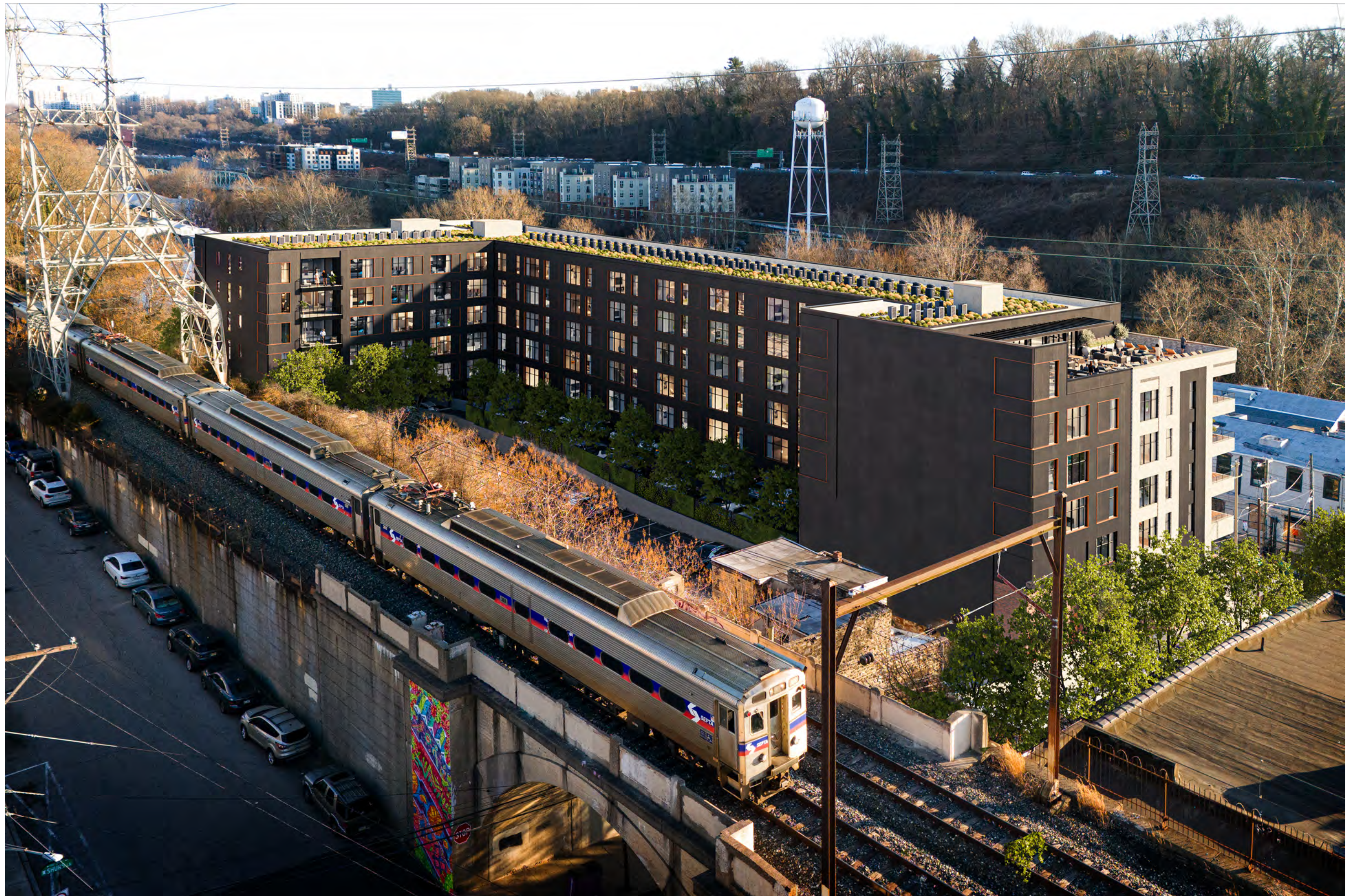
Aerial View looking South
