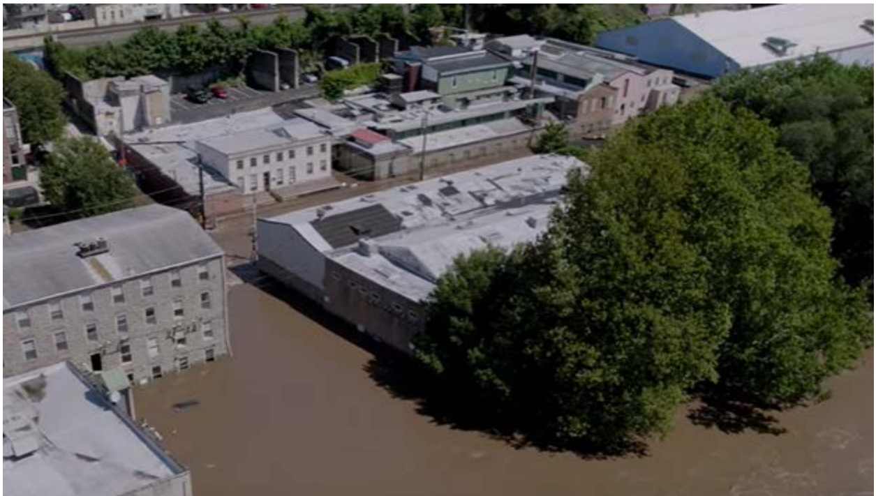
Figure 10. Hurricane Ida flooding in 2021. The photograph shows the water level at the first-floor porch roofline at the office building and mid-way up the large windows in the one-story industrial structure, roughly 10 feet above grade.
