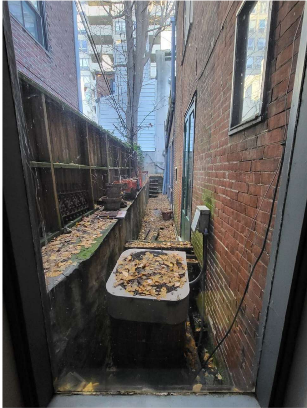
EXISTING CONDITIONS - SIDE YARD SETBACK
