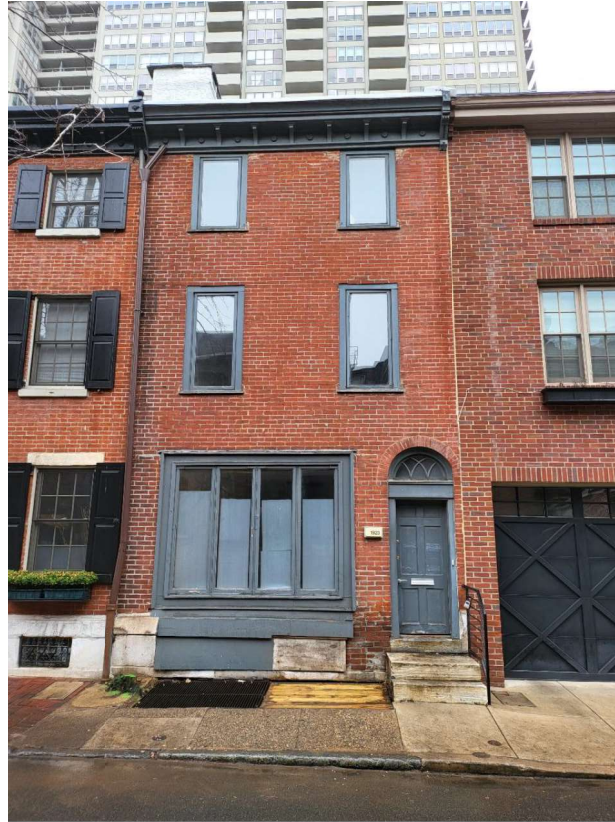
EXISTING CONDITIONS - ACROSS MANNING ST
