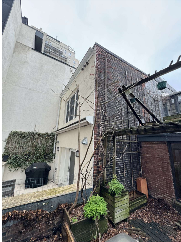
EXISTING CONDITIONS - VIEW EASTWARD FROM 2ND FLOOR REAR
