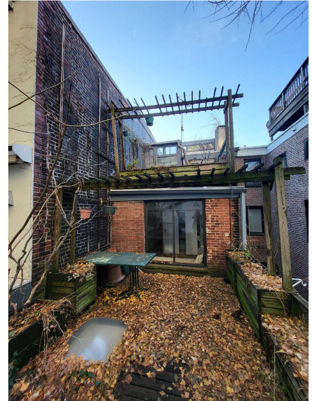
EXISTING CONDITIONS - VIEW FROM 2ND FLOOR REAR ROOF DECK
