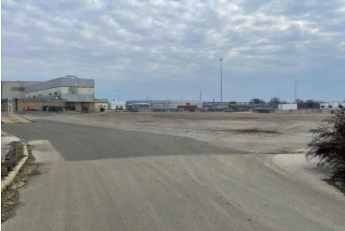
Photo #1: Entrance into site – looking east (to Biosolids Recycling Center)
