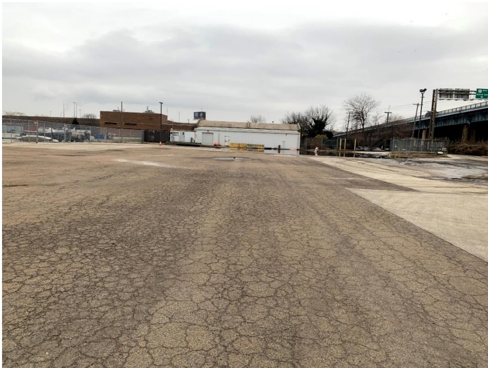
Photo #2: At site – looking west (to PWD Green Stormwater Operations)
