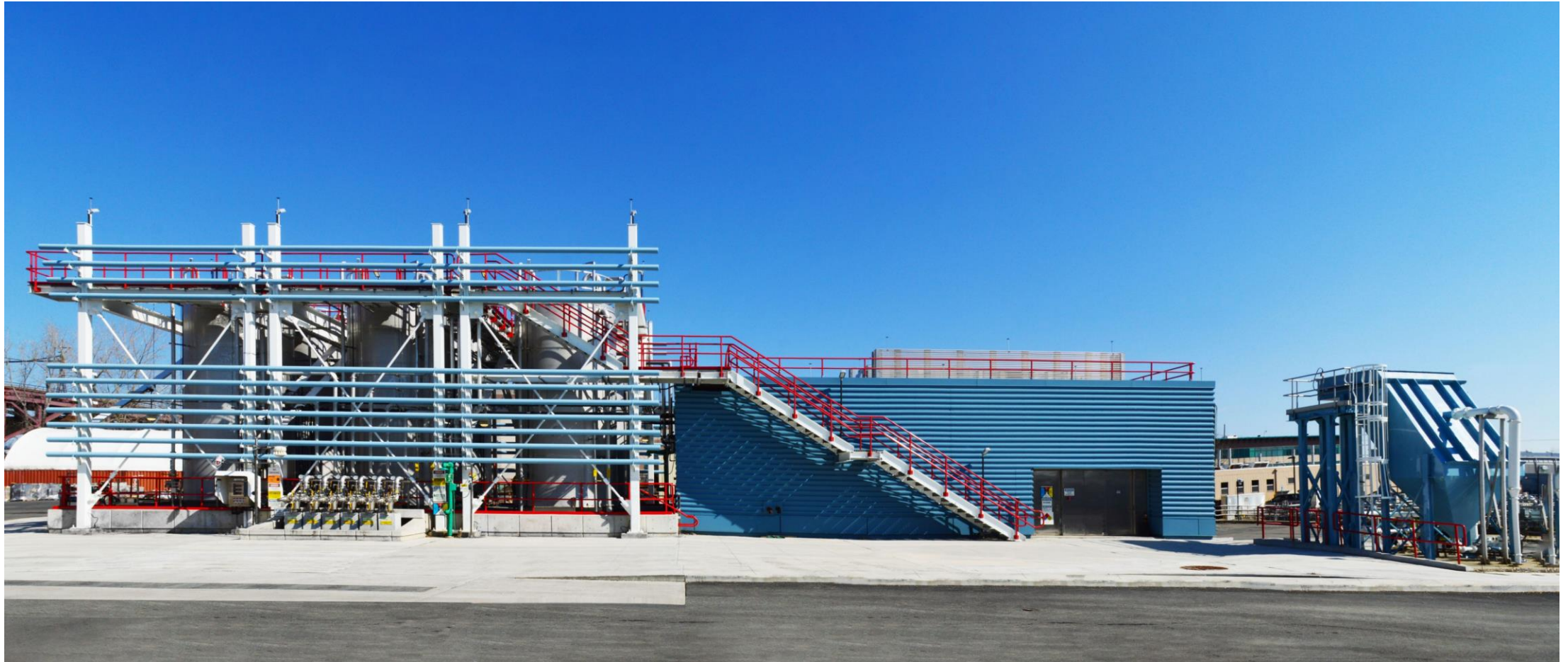
NYC DEP Project: AWT-02, Wards Island, New York
