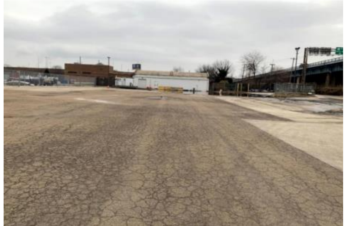
Photo #2: At site – looking west (to PWD Green Stormwater Operations)
