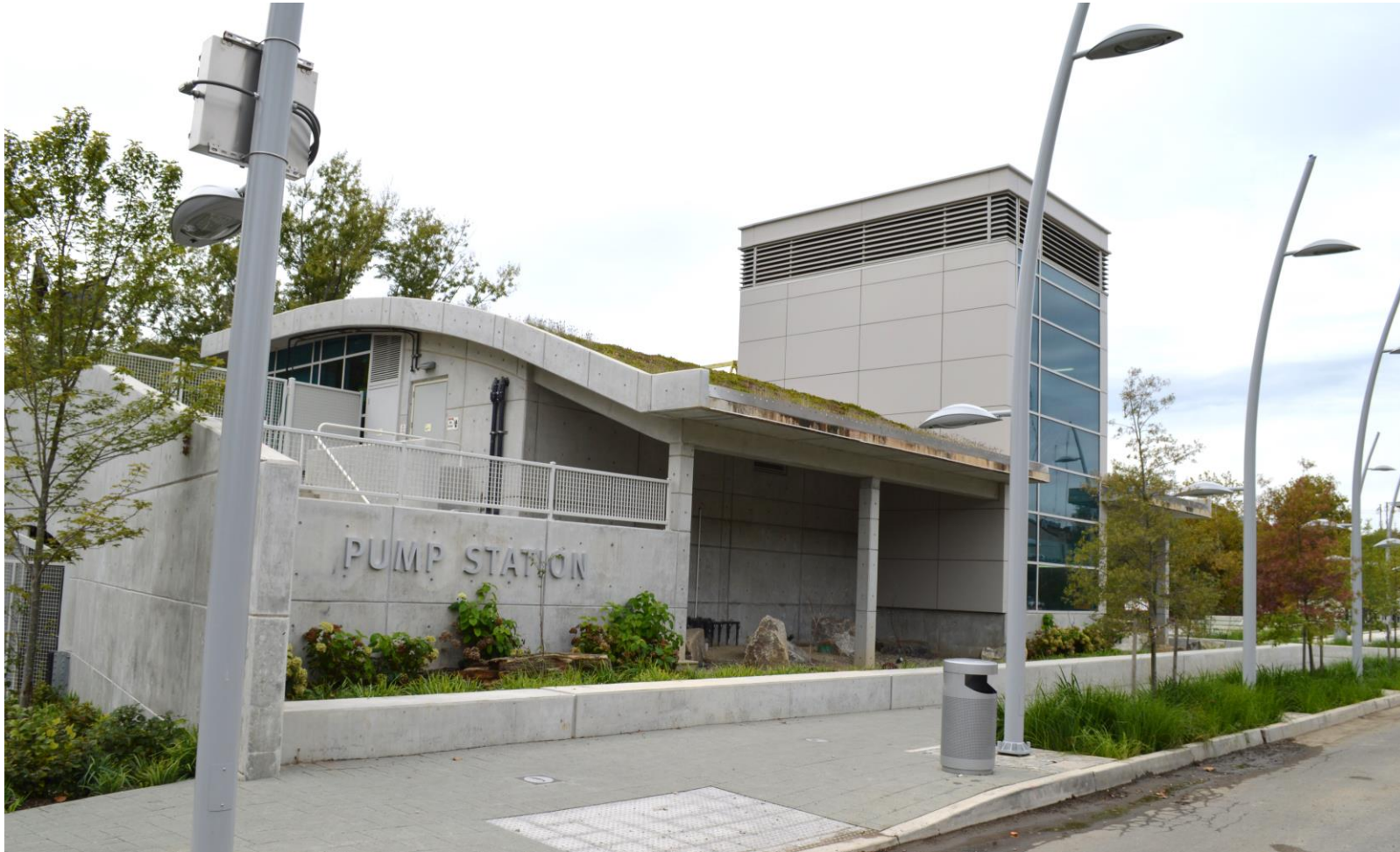
PWD Project: Pump Station, Manayunk, Pennsylvania
