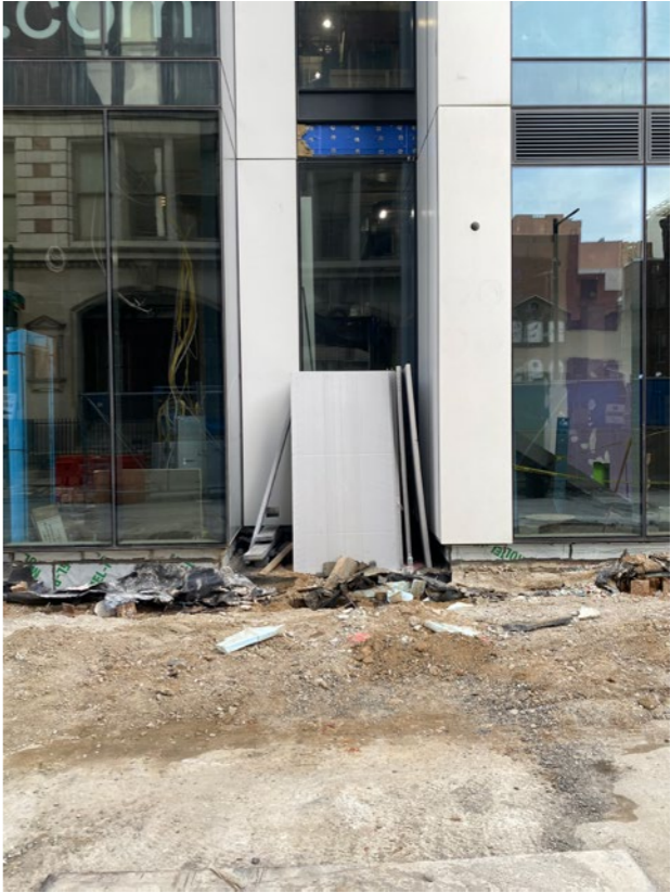
6. Looking directly at the building from across S. 12th Street
