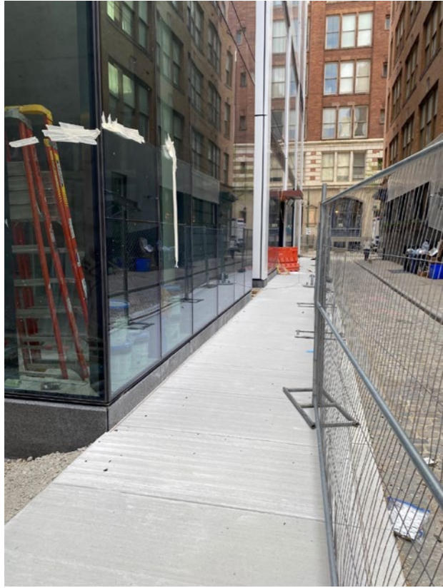
7. Looking up St. James toward S. 12th Street
