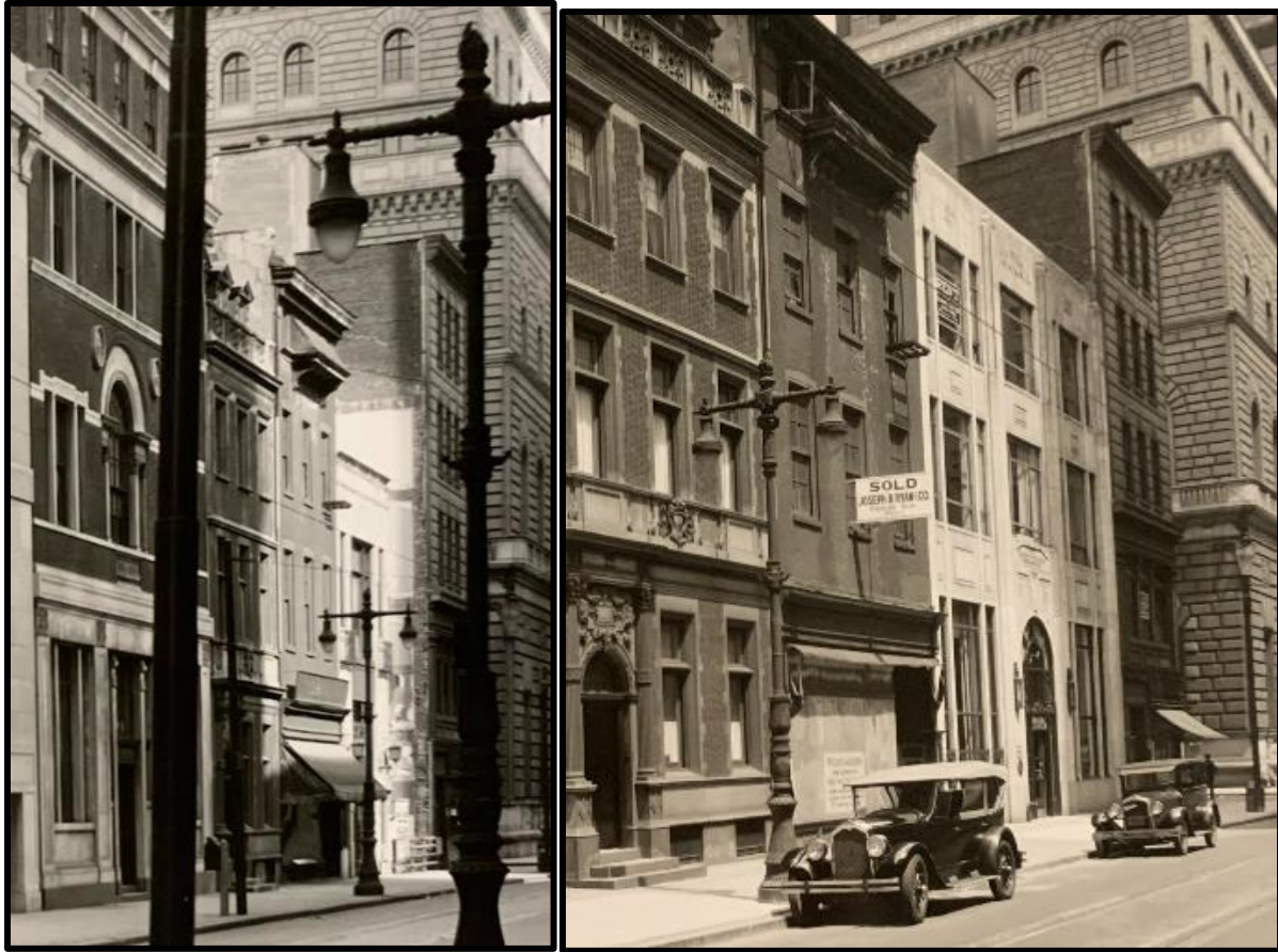
Figure 12. Left: A photograph by Phillip P. Wallace of the 1500 block of Walnut Street with the former two-story building of the City National Bank at 1505 Walnut Street and the recently cleared site of 1503 Walnut Street in October 1930, indicating the initial construction of the subject building. Figure 13. Right: A photograph by Wallace of the 1500 block of Walnut Street with the newly completed City National Bank Building at 1503-05 Walnut Street in May 1932. Source: Boies Penrose Collection, Box 23, Historical Society of Pennsylvania.
