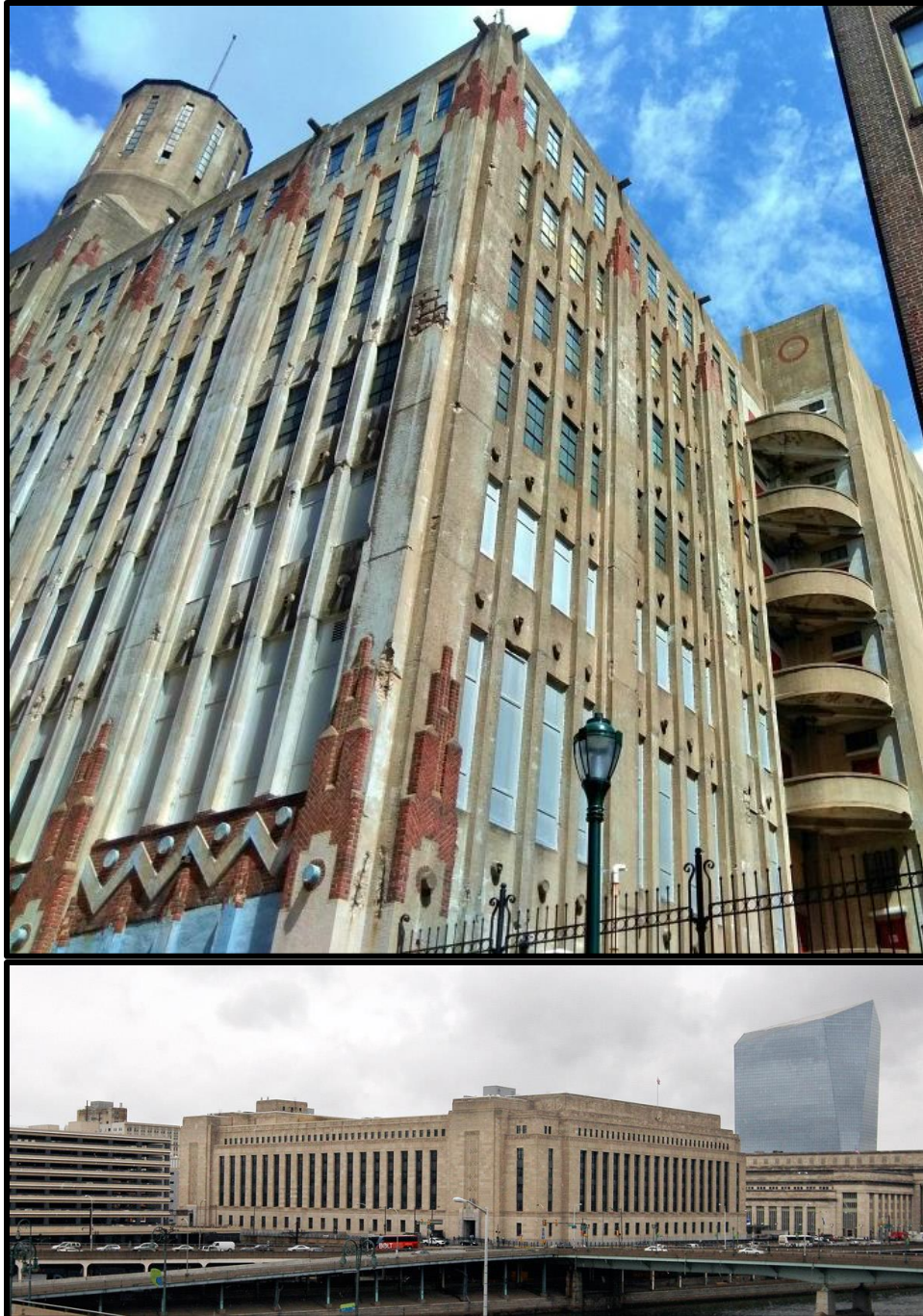
Figure 20. Top: The Lasher Printing Co. at 1309 Noble Street. Source: The Rail Park And My Attraction To Industrial Design [ Being Ron ] (triloquist.net) . Figure 21. Bottom: The U.S. Post Office Building (1930) and 30 th Street Station (at right, completed 1933). Source: The Philadelphia Inquirer .
