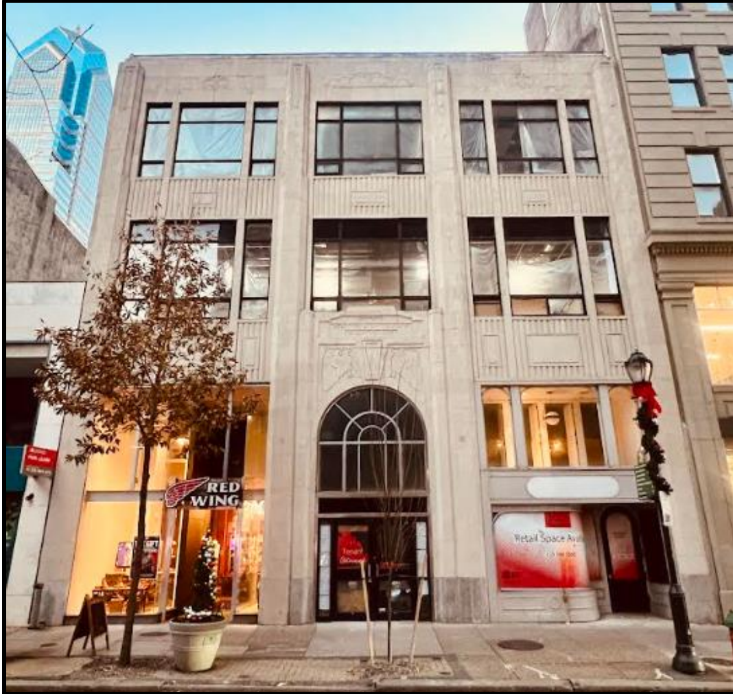
Figure 3. The primary (south) elevation of the subject property prior to the collision, in July 2023, of a bus with the left portion of the first-floor facade. Source: Oscar Beisert.
