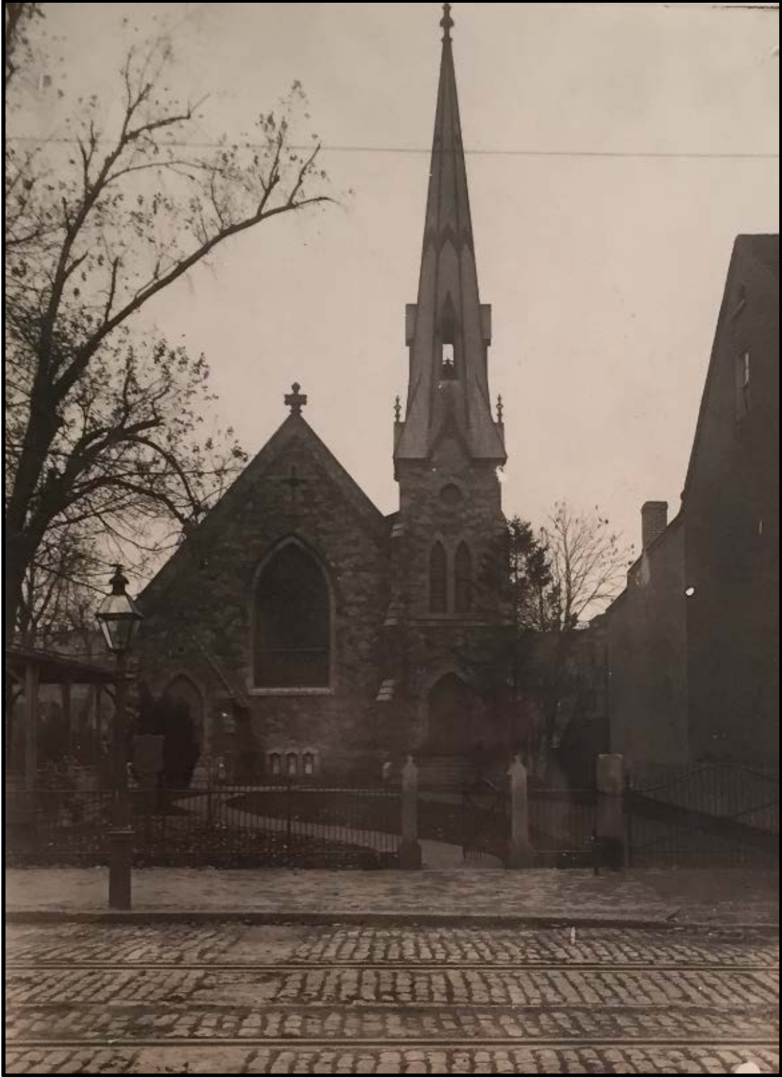
Figure 20. St. Stephen's M. E. Church, 5209-13 Germantown Ave, Primary (Southwest) Elevation, ca.1880. Source: GHS.
