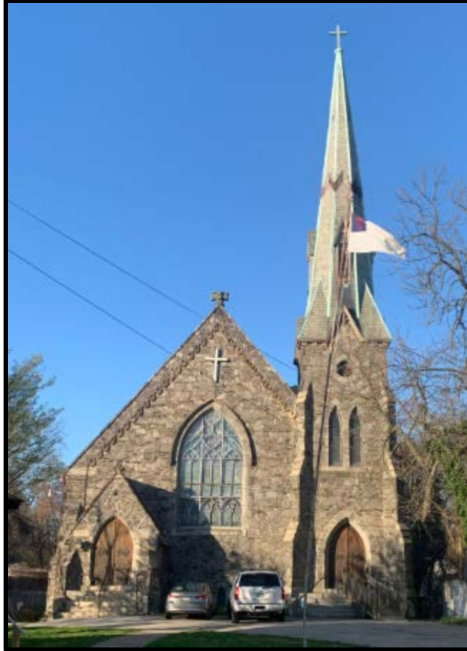
Figure 5. St. Stephen's M.E. Church, 5209-13 Germantown Avenue, Primary (Southwest) Elevation. Source: Oscar Beisert, 2023.
