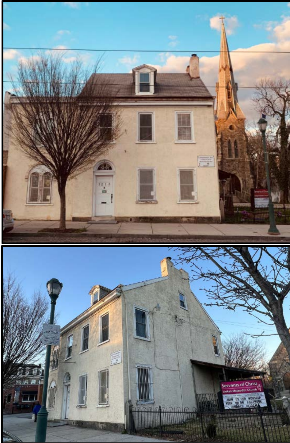
Figure 15. Top: The primary (southwest) elevation of the Fraley House, aka the Parsonage of St. Stephen's M. E. Church. Source: Oscar Beisert, 2023. Figure 16. Bottom: The primary (southwest) and side (southeast) elevations of the Fraley House, aka the Parsonage of St. Stephen's M. E. Church. Source: Oscar Beisert, 2023.
