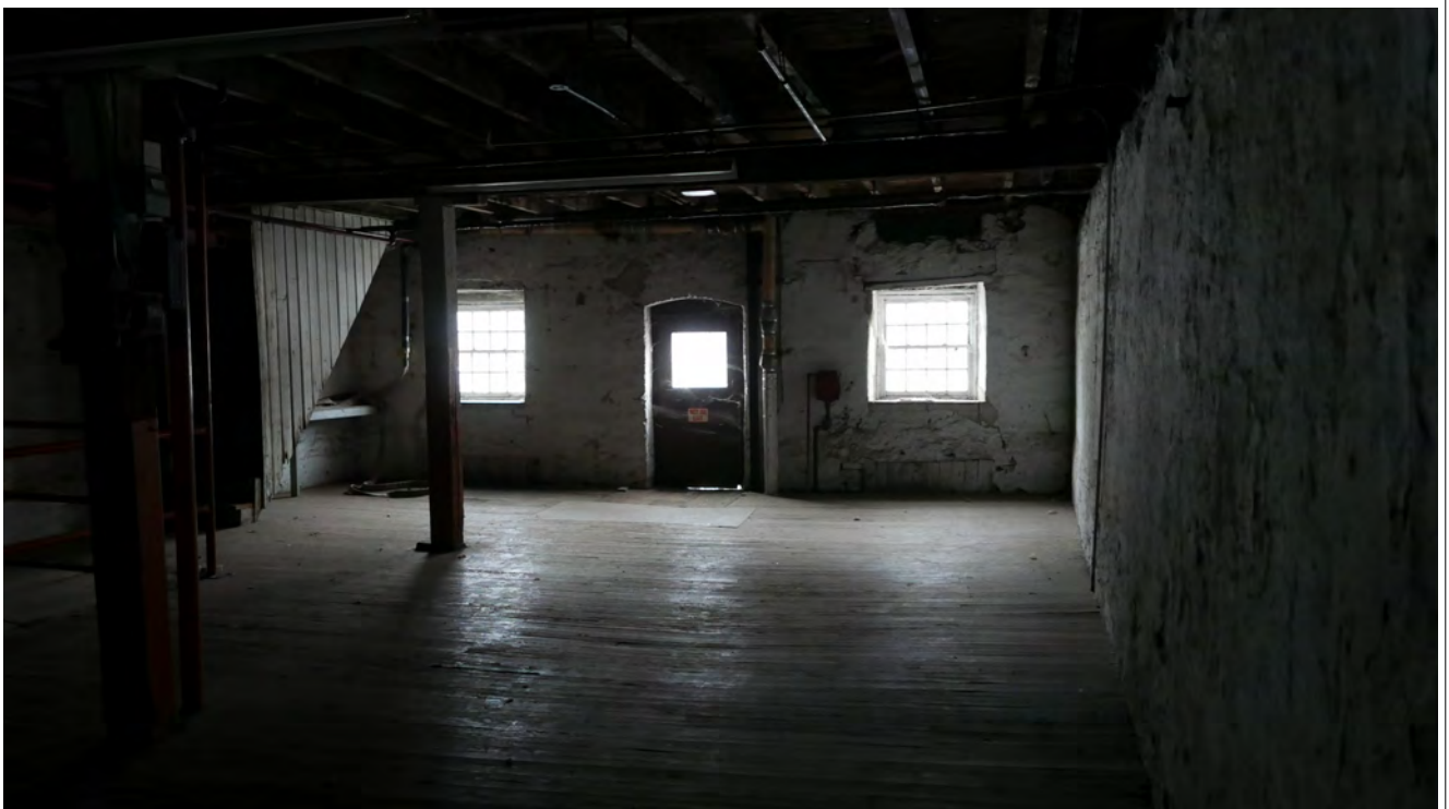
Illustration 9: Structure 7 second floor. Also a third floor above
