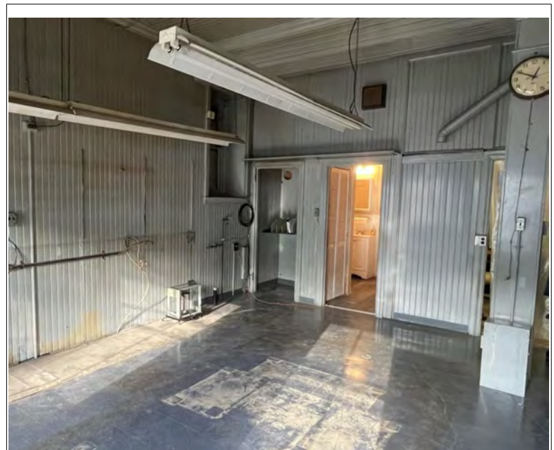
Illustration 13: Pre-1850 Historic Hotel Building 2nd Floor Office with 12' Ceilings
