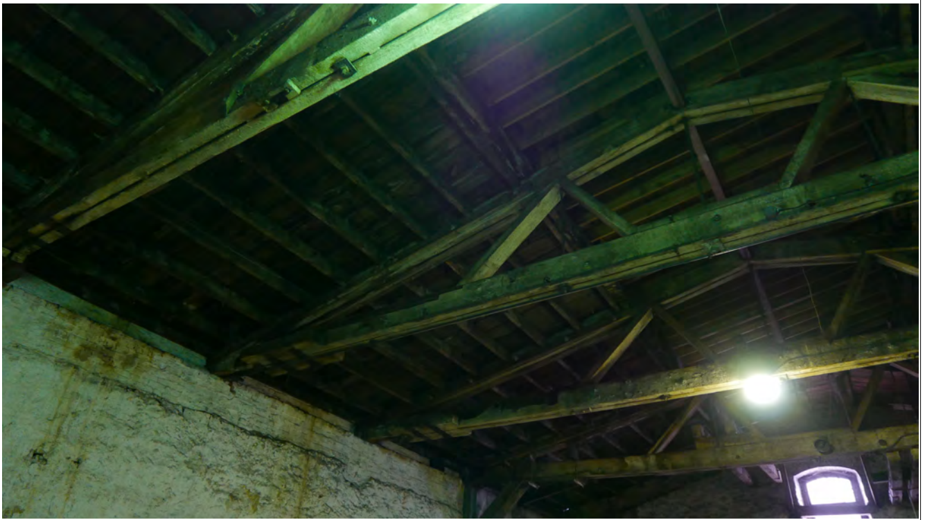
Illustration 10: Structure 8 Roof and Trusses
