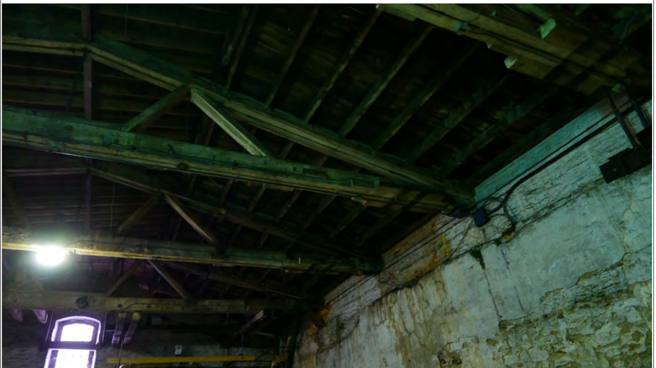
Illustration 11: Structure 8 Roof and Trusses
