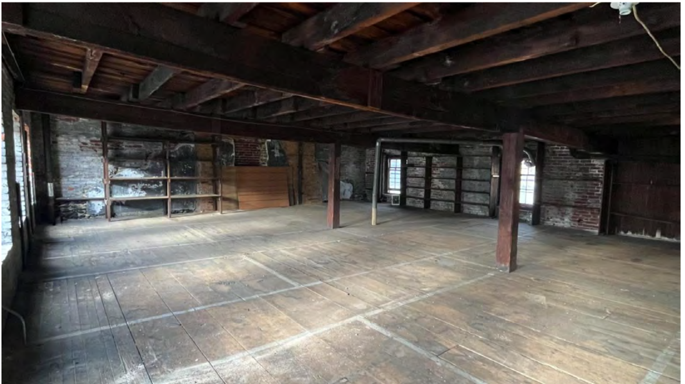
Illustration 12: Pre-1850 Historic Hotel Building 3rd Floor
