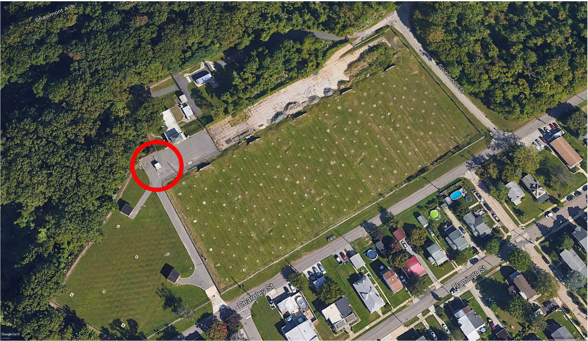
Figure 5 – ROX North Aerial View
