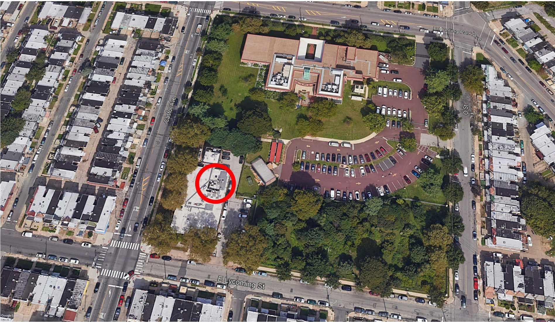
Figure 3 – LAB North Aerial View
