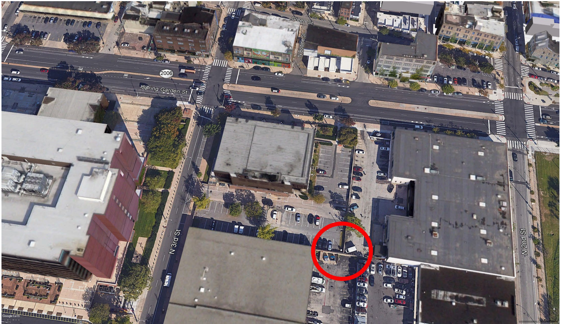
Figure 13 – FAB North Aerial View
