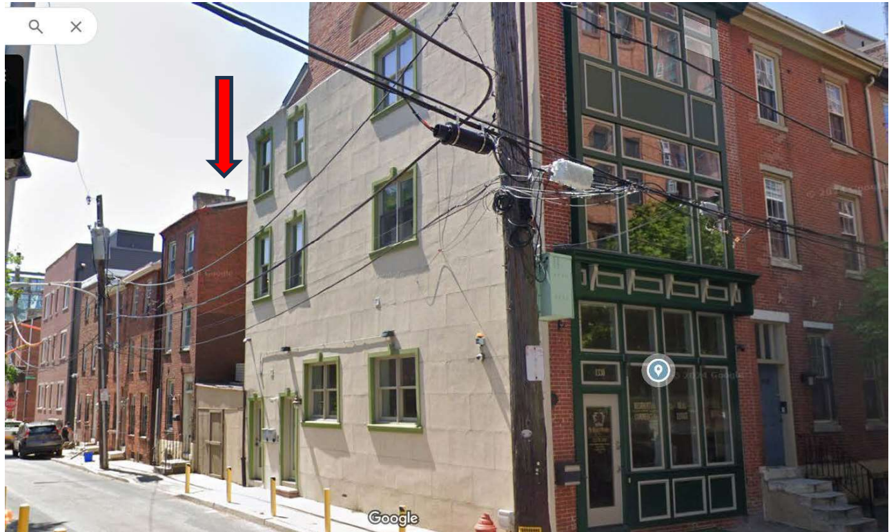
Figure 1. View from Juniper and Lombard Streets, showing the existing garage and three-story building at 502-04 S. Juniper Street, which the Historical Commission approved for demolition owing to a finding of financial hardship.
