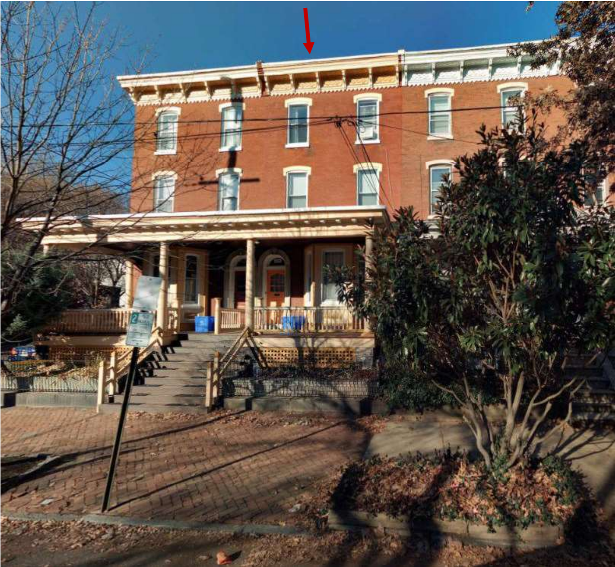
Figure 2: View of front façade of 3629 Hamilton St from Hamilton St:
