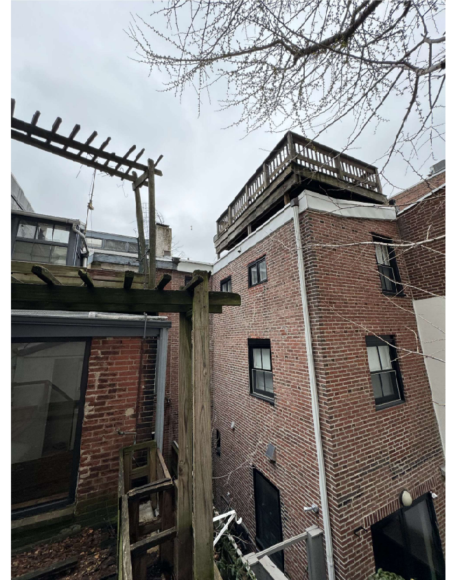
EXISTING CONDITIONS - VIEW WESTWARD FROM 2ND FLOOR REAR
