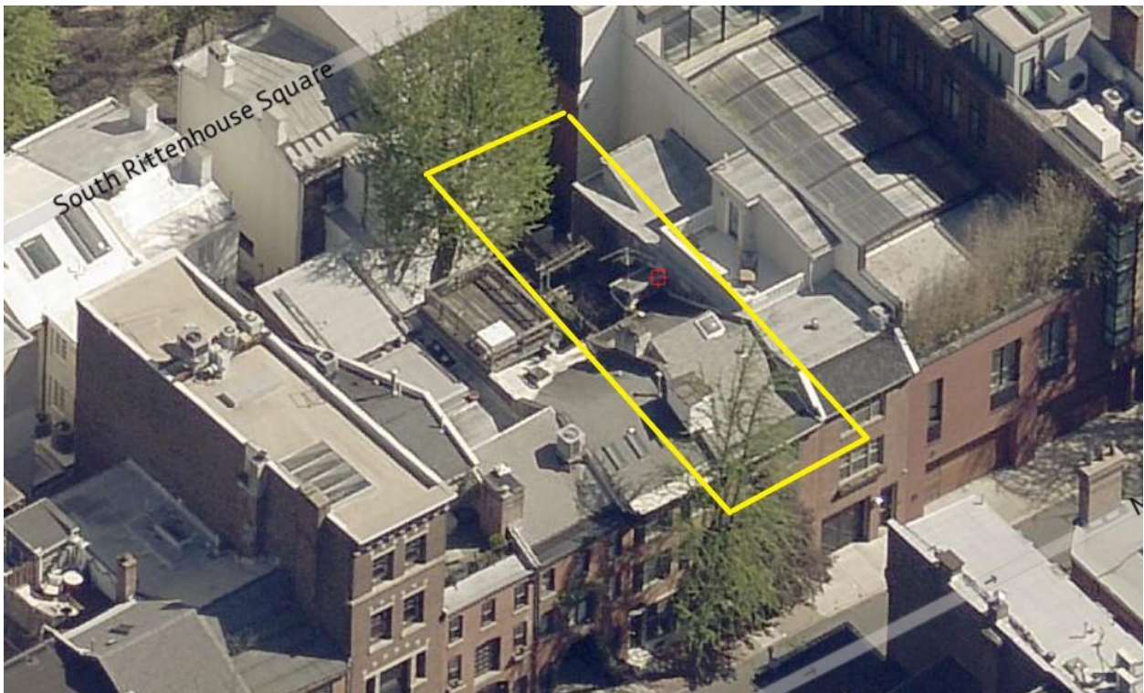
Figure 2: Aerial view looking northeast at 1923 Manning Street roof.
