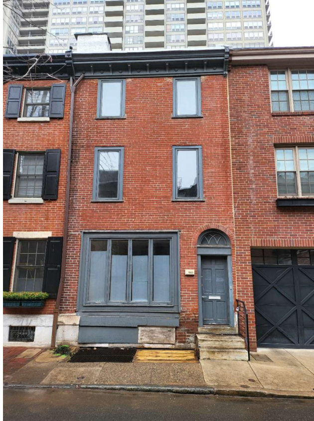
EXISTING CONDITIONS - ACROSS MANNING ST
