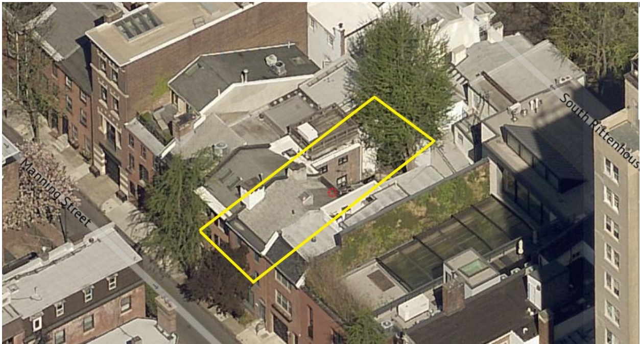
Figure 1: Aerial view looking northwest at the 1923 Manning Street roof.
