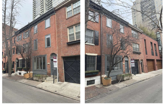
2 PHOTO OF EXISTING STREET CONDITIONS 2-100 NTS
