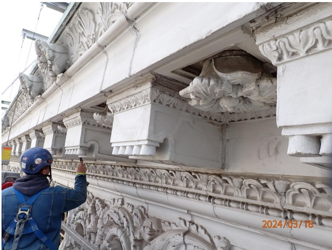
Photograph 6 – Close-up view of terra cotta flower units between dentil units.
