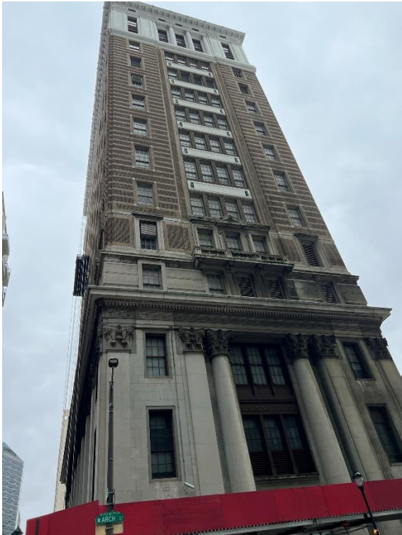
Photograph 2- Overview of south elevation.
