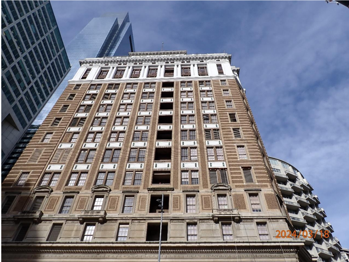
Photograph 3 – Overview of east elevation.
