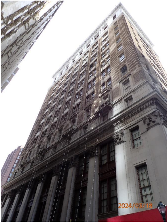
Photograph 1 – Overview of west elevation.
