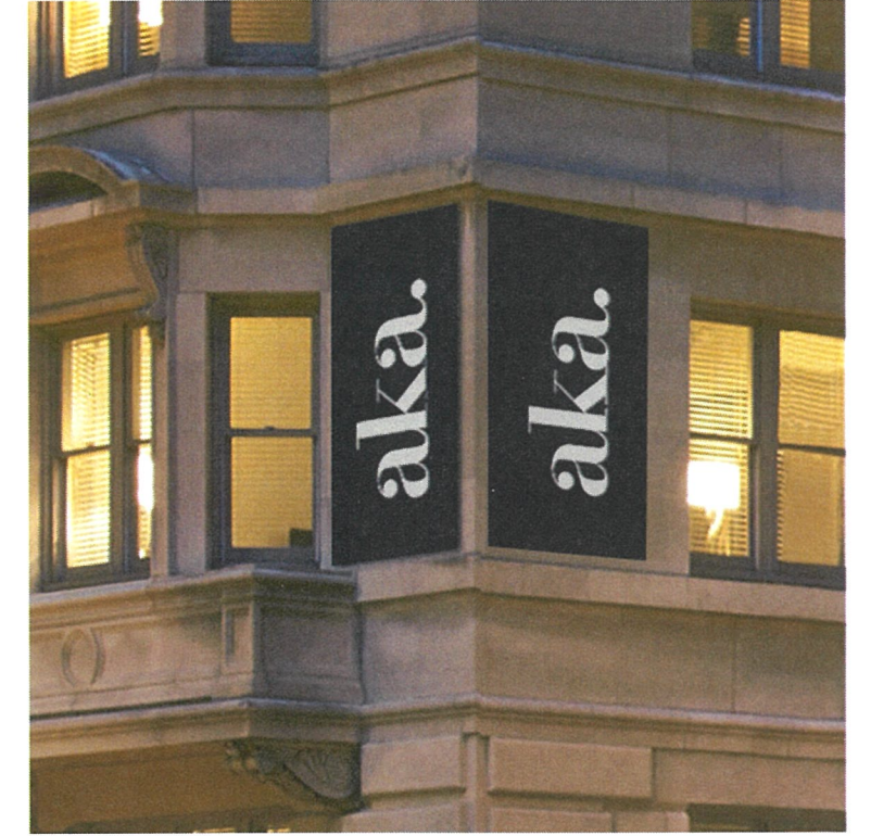
3rd Floor Corner Sign
