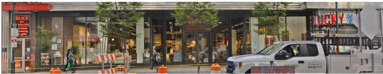
2023 – Dark window frames, darkened glass, small doors, and asymmetrical shop window
