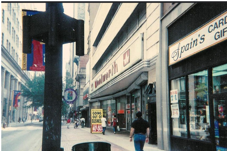
Woolworth's Store 1997 at time of going out of business sale with anti-theft grills and colonial doorway on west end of façade. 24
