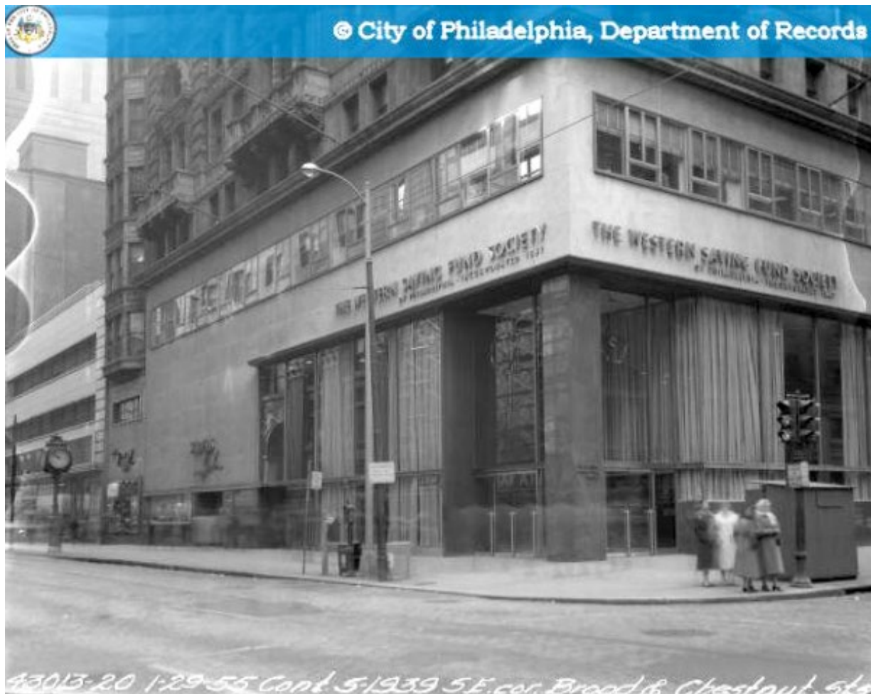
Three story yellow sandstone base with polished brown granite corner pier for Western Savings Fund Society offices, Woolworth store to the left, January 29, 1955 PhillyHistory.
