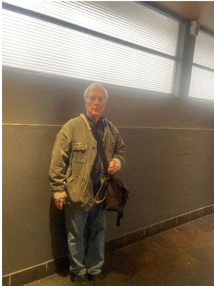
Present window 71" heights above floor with inoperable sash
