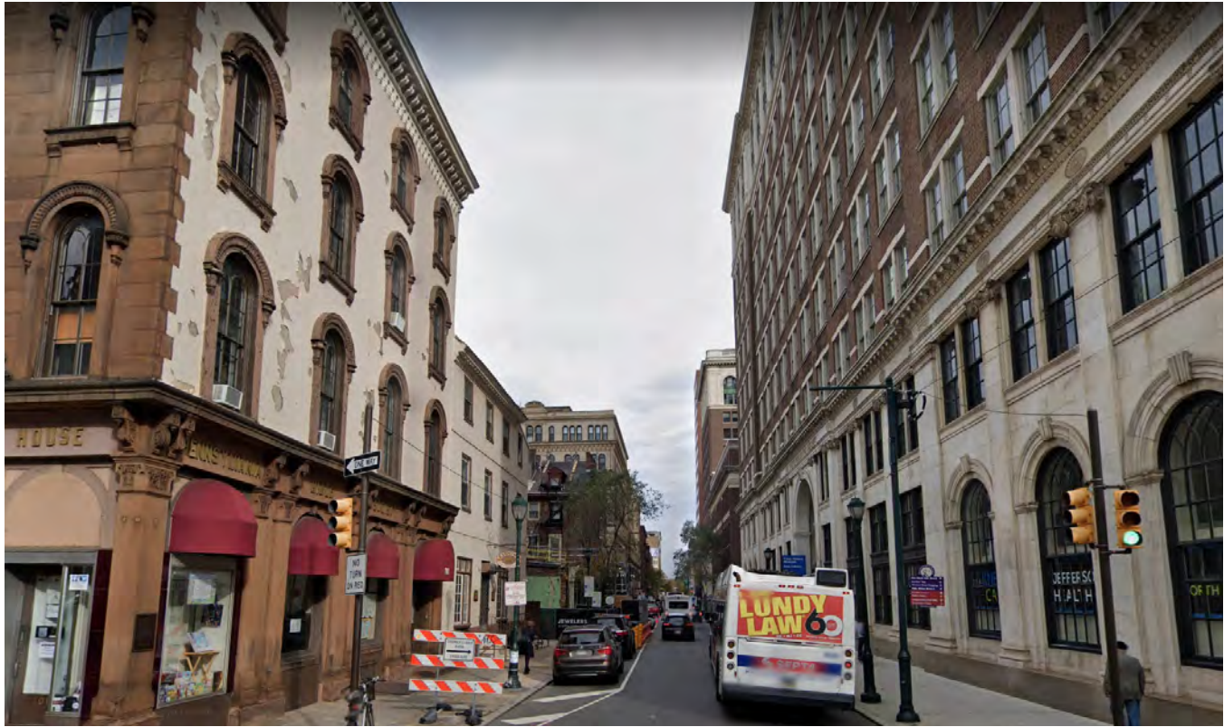
3 Looking North on 7th Street
