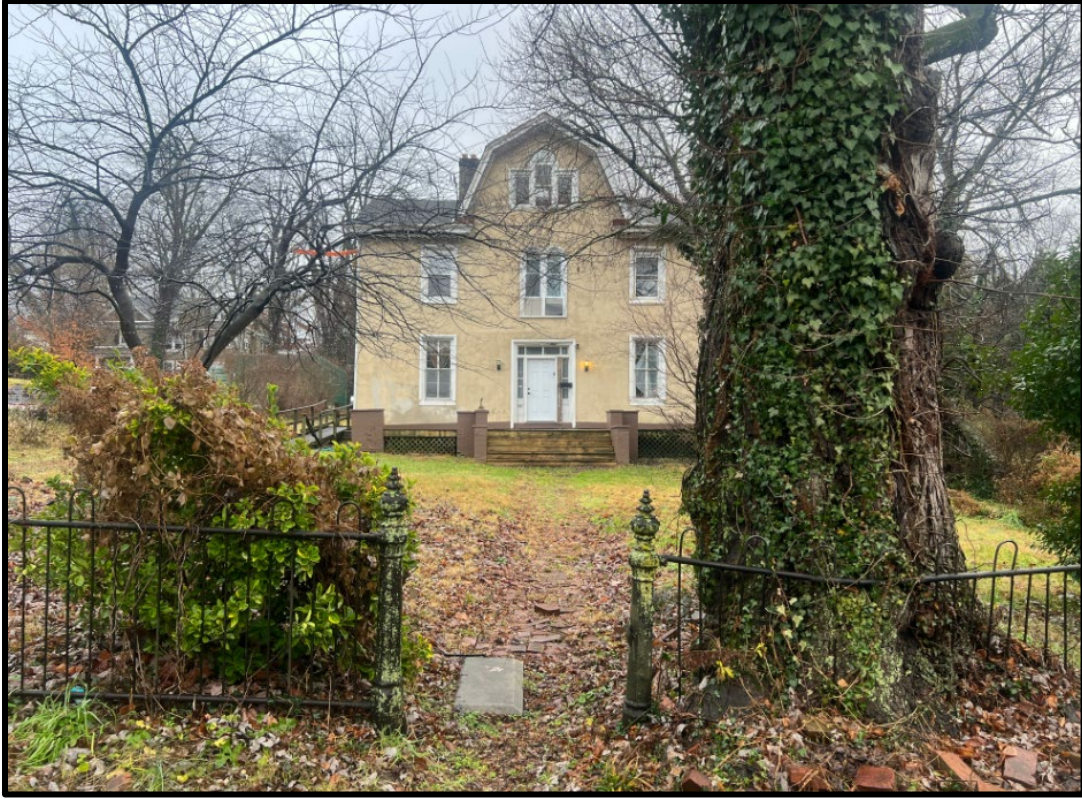
Figure 3. The Smith-Steel-Humphreys House, 424 E. Woodlawn Avenue, Primary (Northwest) Elevation. Source: Oscar Beisert, 2023.
