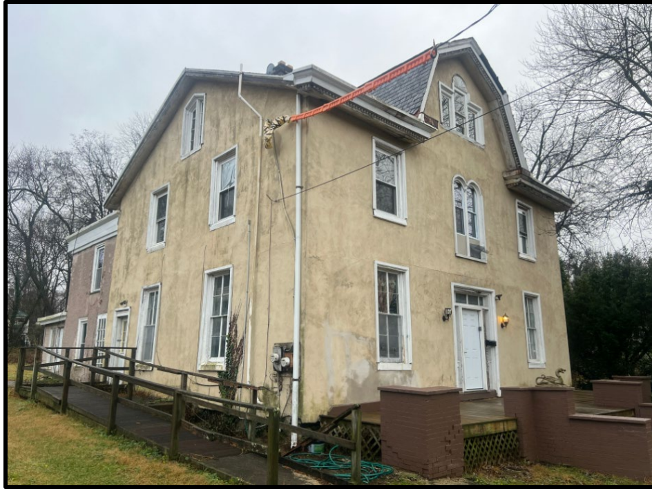
Figure 6. The Smith-Steel-Humphreys House, 424 E. Woodlawn Street, Primary (Northwest) and Side (Northeast) Elevations. Source: Oscar Beisert, 2023.
