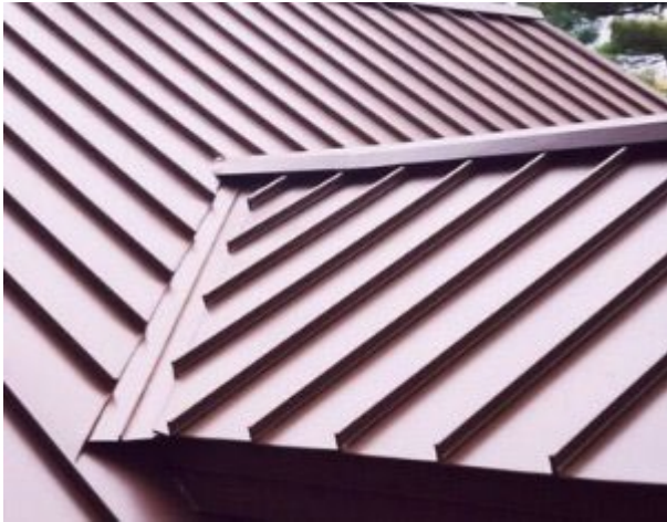
Standing Seam Metal Roof
