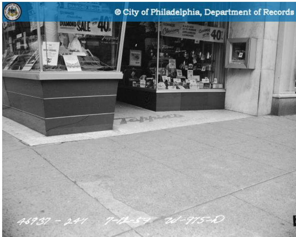
Figure 29: A 1959 photo shows the entrance to Tappin's at street level.
