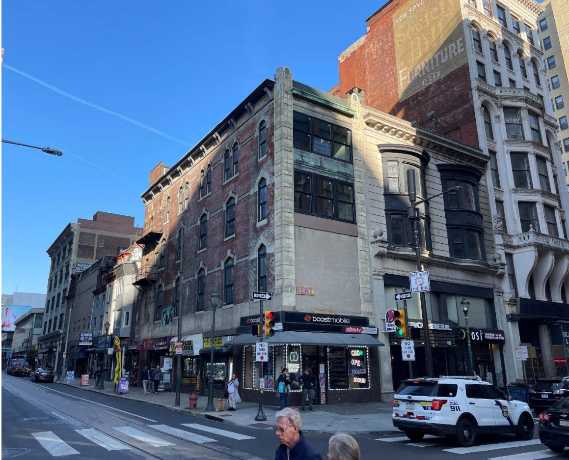
Figure 4: View of 1039 Chestnut Street, looking Northeast. Photo by author, October 2023.
