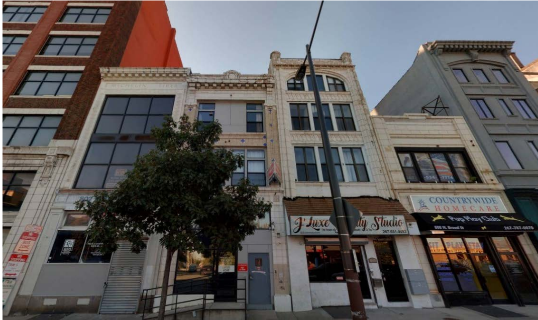
Figure 46: 802, 804, 806, and 808 North Broad Street are examples of the Commercial Style.
