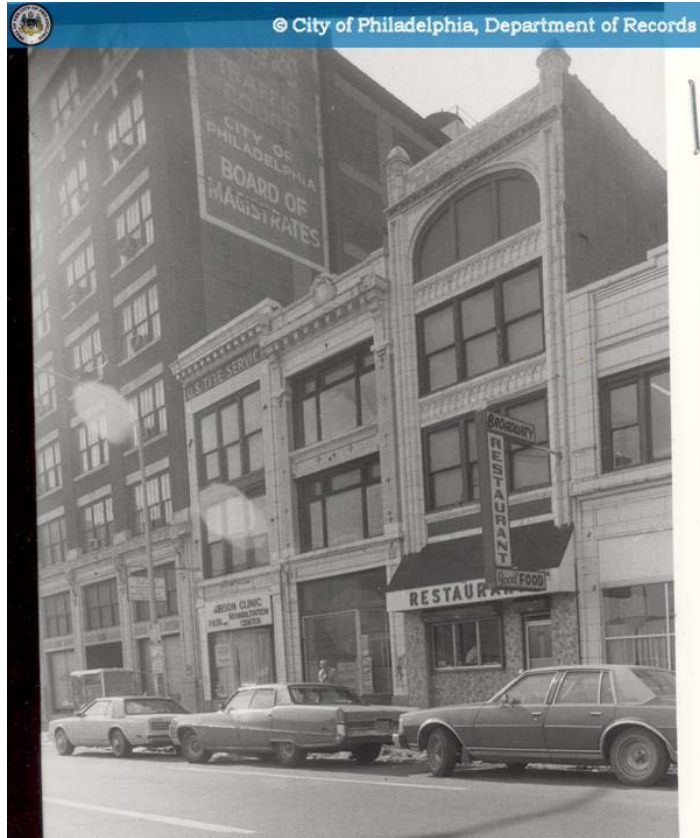
Figure 47: 802, 804, 806, and 808 North Broad Street. The date of the photograph is unknown, but it was taken after the top two floors of 808 were removed in 1941.
