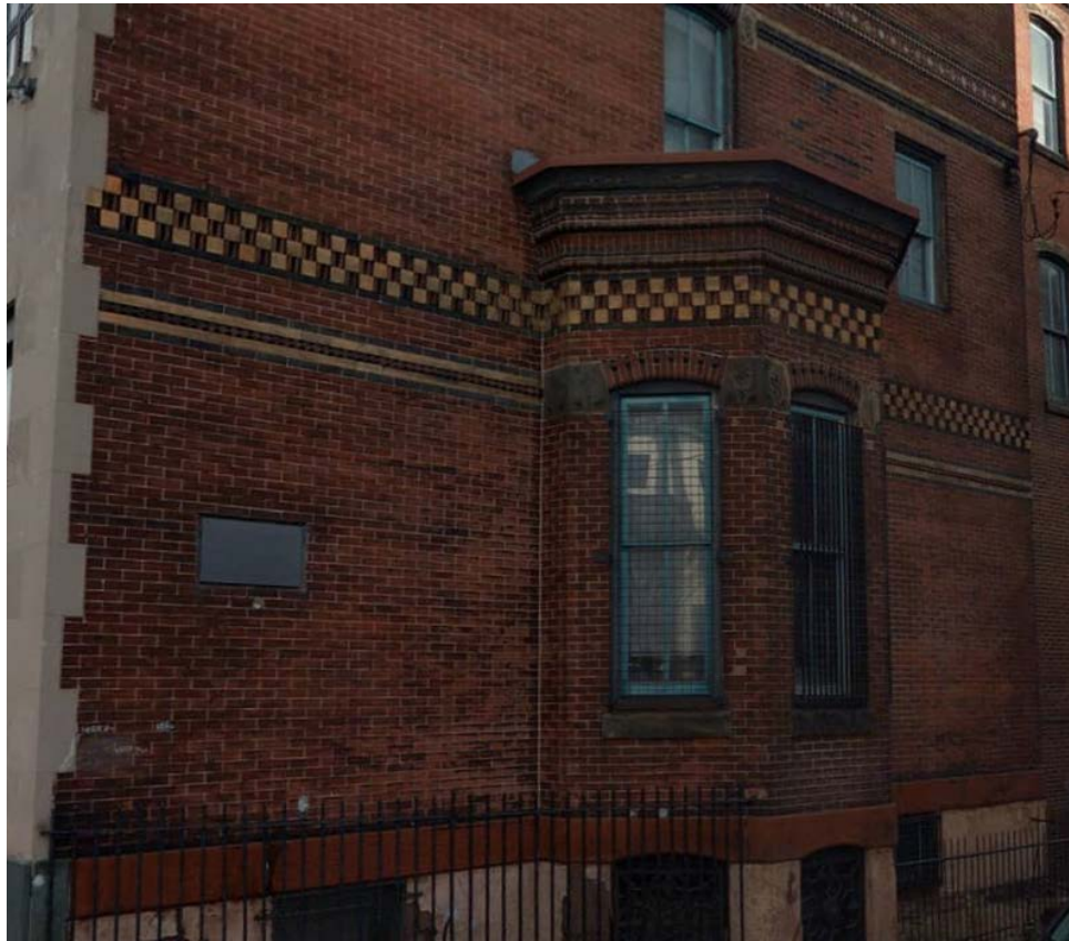
Figure 35: Polychrome brick on the Fitzwater elevation of 731 S. Broad Street. Image from Cyclomedia.phila.gov
