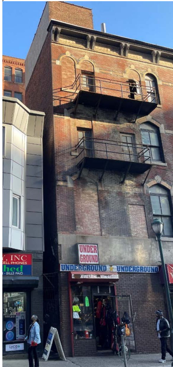
Figure 15: A narrow alley runs along the rear of 1039 Chestnut Street. The narrow aperture and debris in the alley make it difficult to photograph the North facade.
