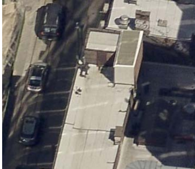
Figure 16: Aerial view of the utility room/pilot house on the roof of 1039 Chestnut Street and the party wall with 1037 Chestnut Street (right). Image from Pictometry.phila.gov.
