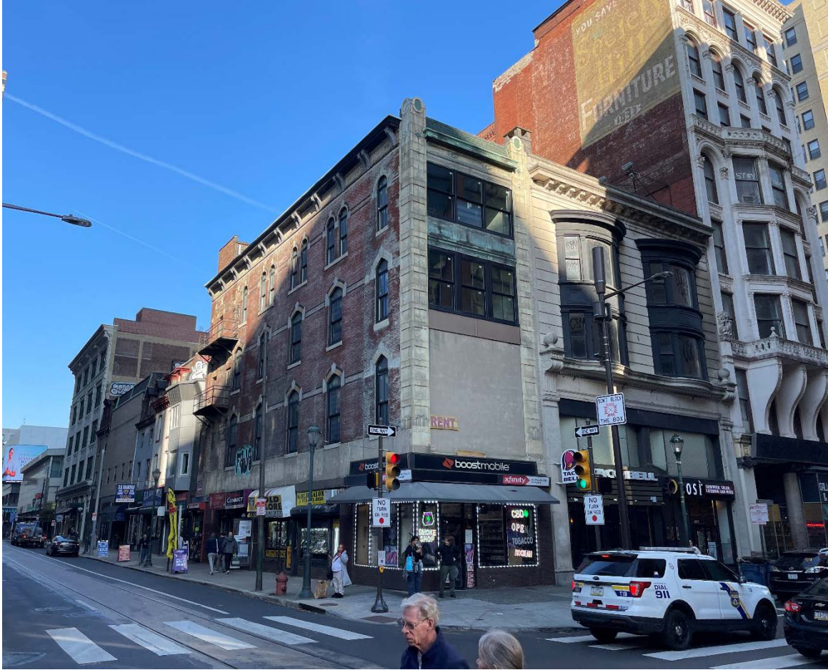
Figure 1: View of 1039 Chestnut Street, looking Northeast. Photo by author, October 2023.
